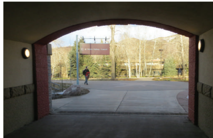
Figure 2.2: Bicycle and Pedestrian Underpass - Aspen
