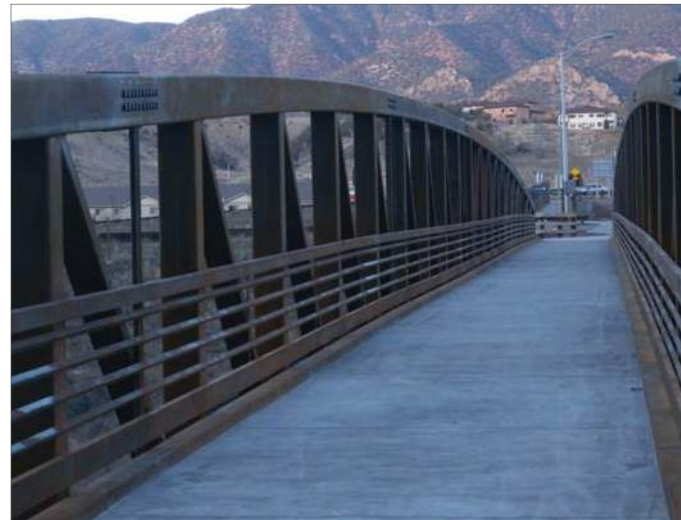
Figure 3.5: Shared-Use Path Bridge over I-70/Colorado River/Railroad - New Castle
