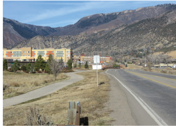
Figure 2.11: Shared Use Path along Roadway - Glenwood Springs
