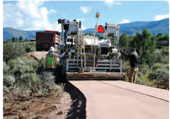
Preparing a dual surface above Woody Creek.
