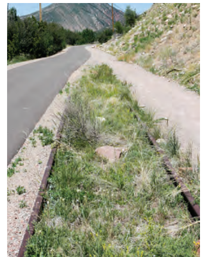
Section of rail remaining in Woody Creek.
