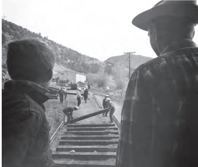
Replacing ties and rails in 1967. Aspen Historical Society photo
