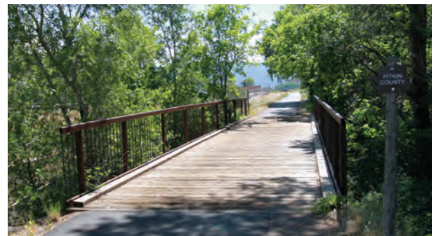
Emma Bridge at the Pitkin County line.
