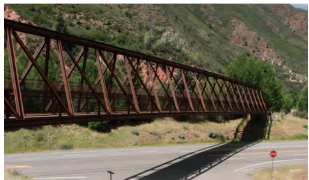
The Wingo bridge over Highway 82.
