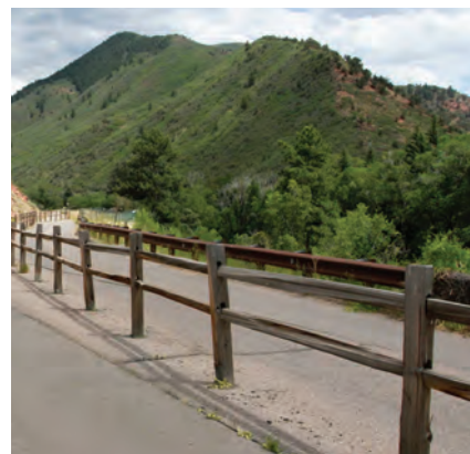
Two-rail, split rail fence is standard along the Rio Grande Trail.
