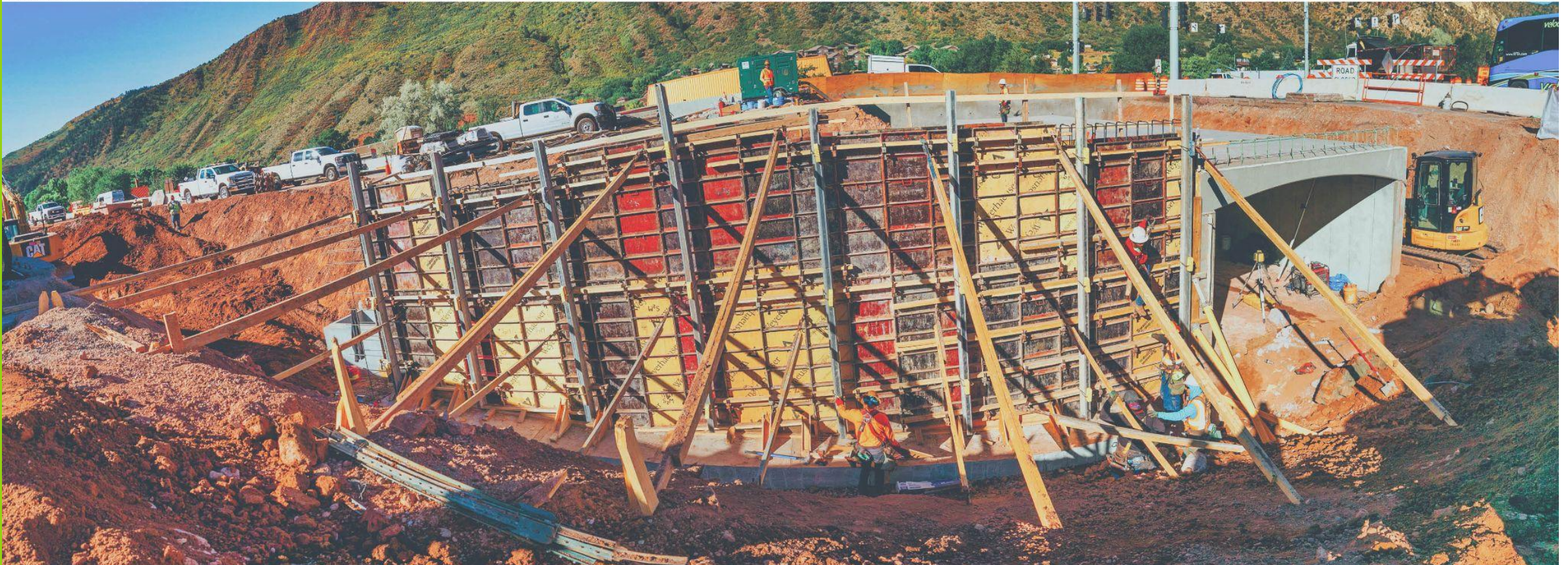
East side portal of the SH82 tunnel and wall forming
