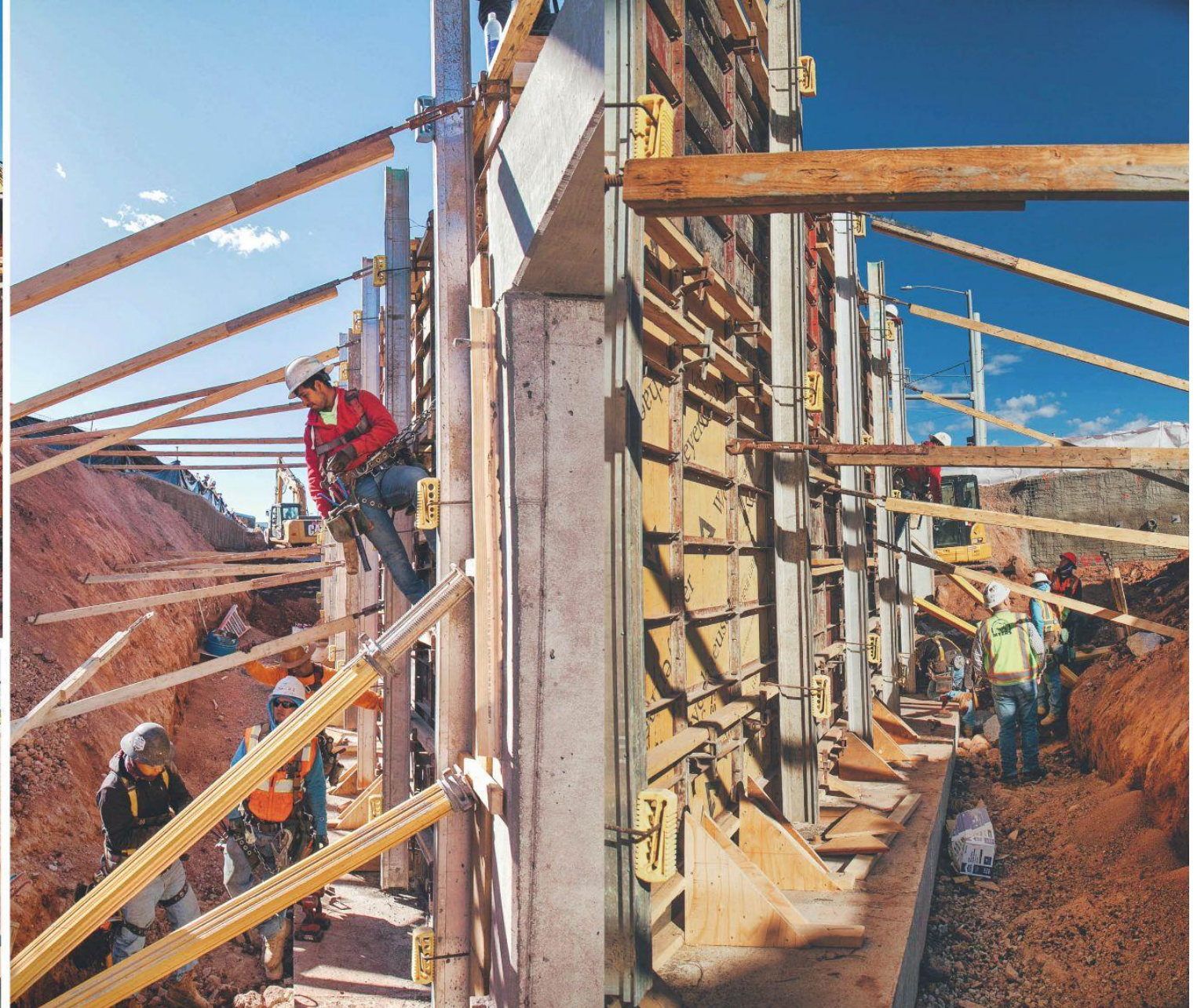
Retaining walls along the access trail to the east portal
