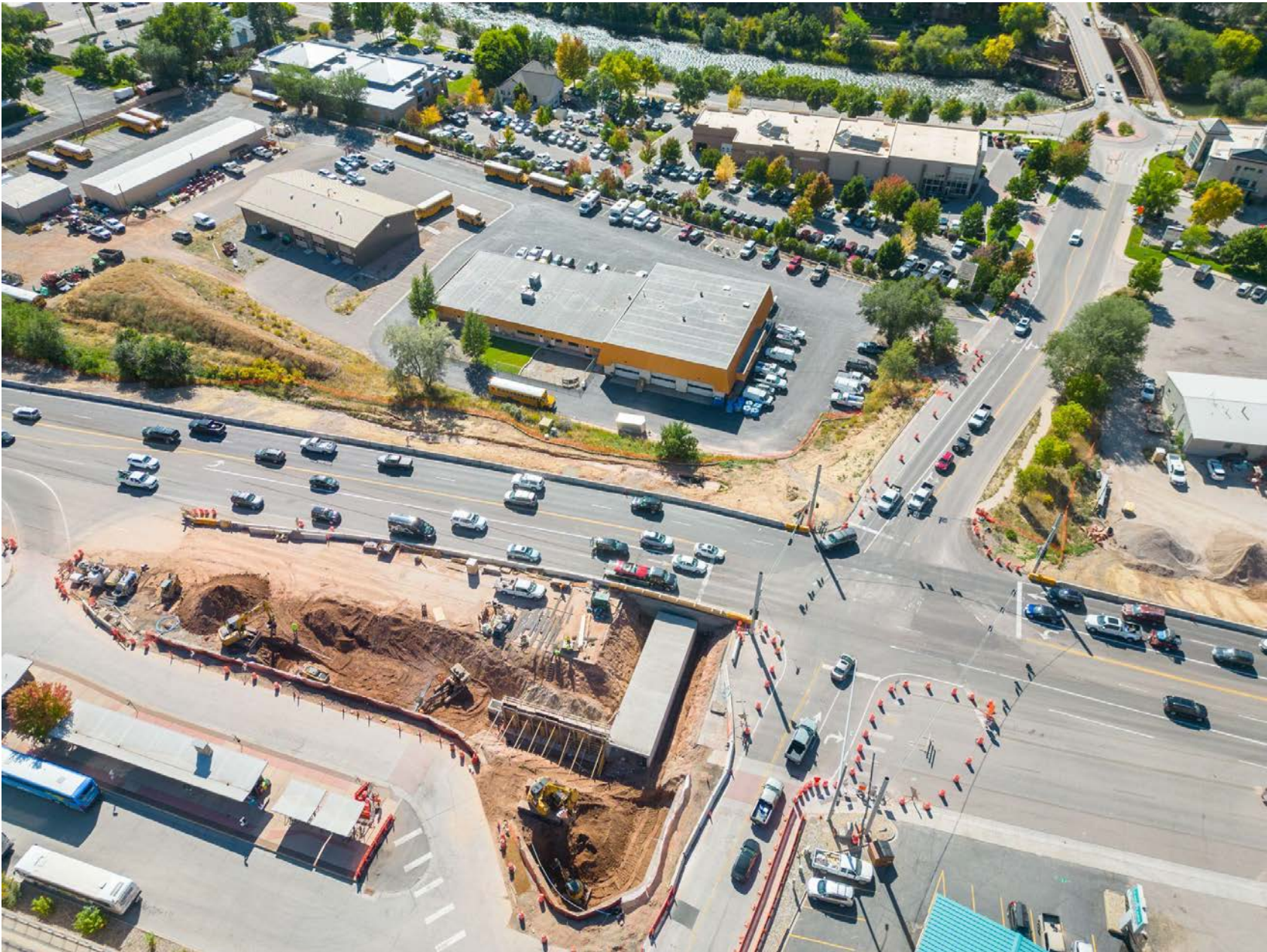
Drone photo from 27th Station and SH 82 construction site
