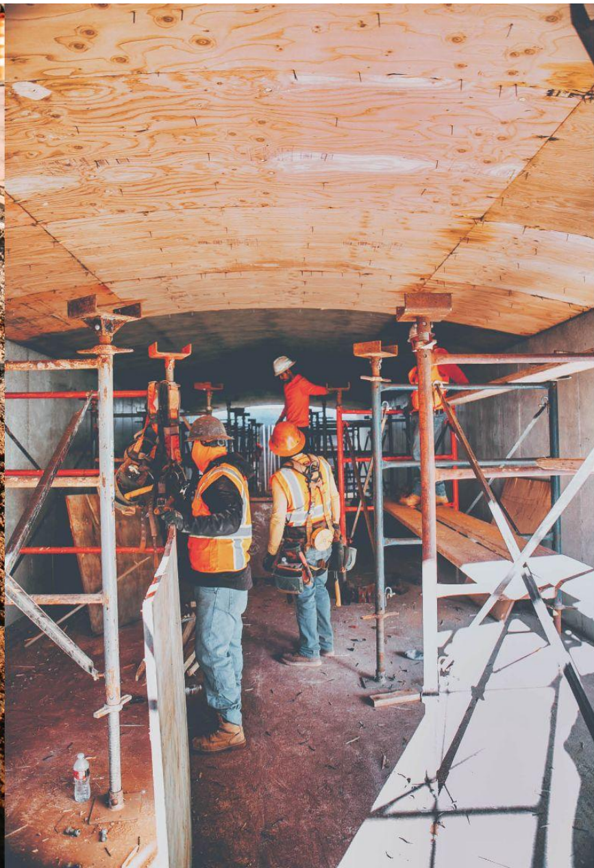
Shoring for excavation and interior tunnel ceiling forming
