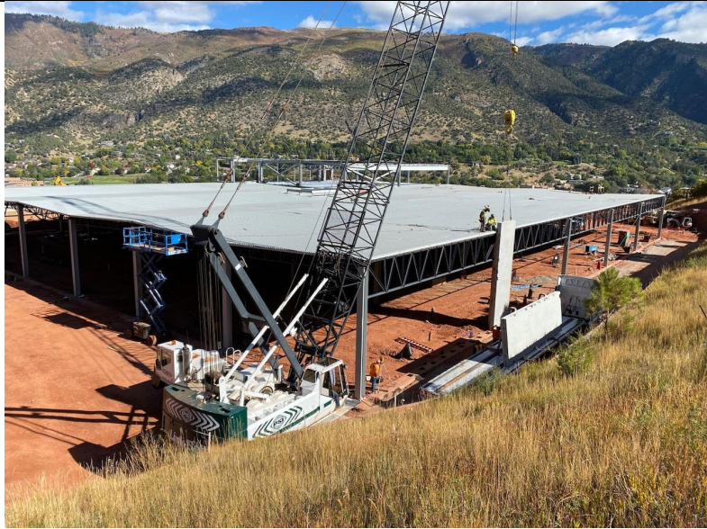
Wall panels being tilted in place
