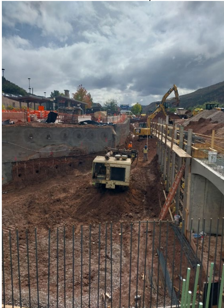
East side of HWY 82 underpass at 27 th Street Station
