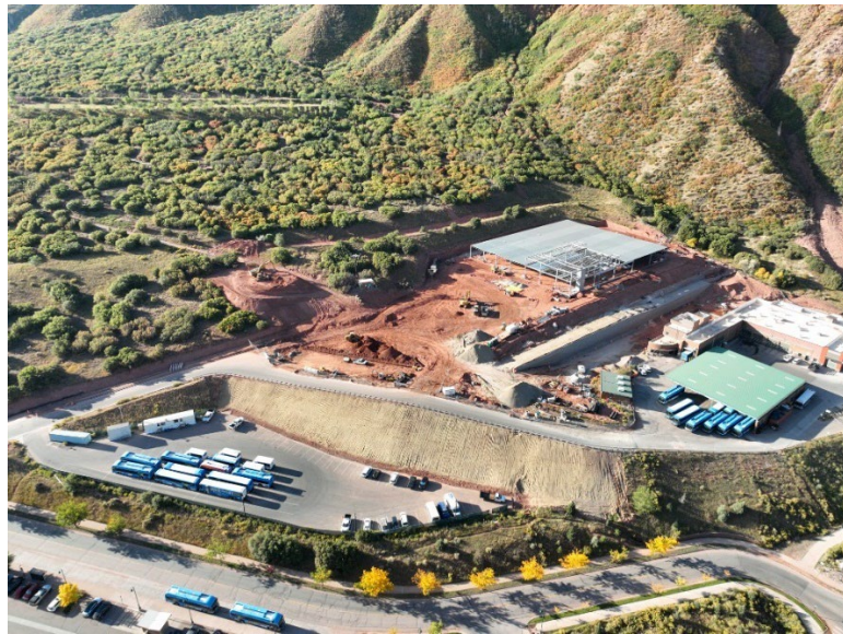
Aerial view of GMF construction site
