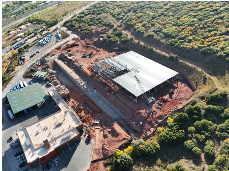
Aerial view of GMF construction site
