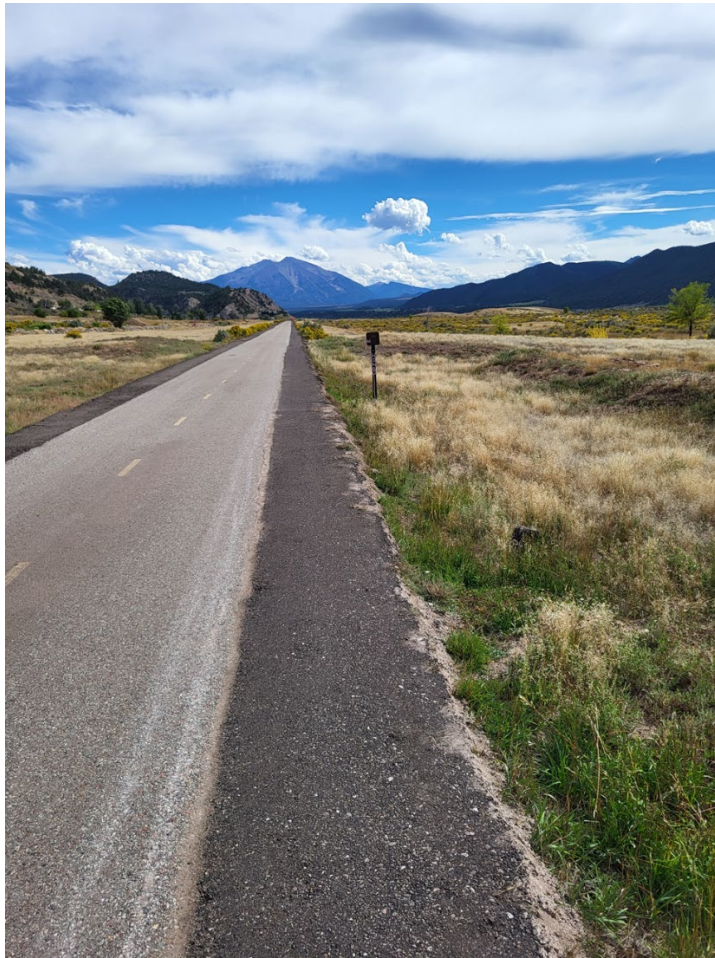
Photo – completed gravel shoulders (compacted recycled asphalt pavement)
