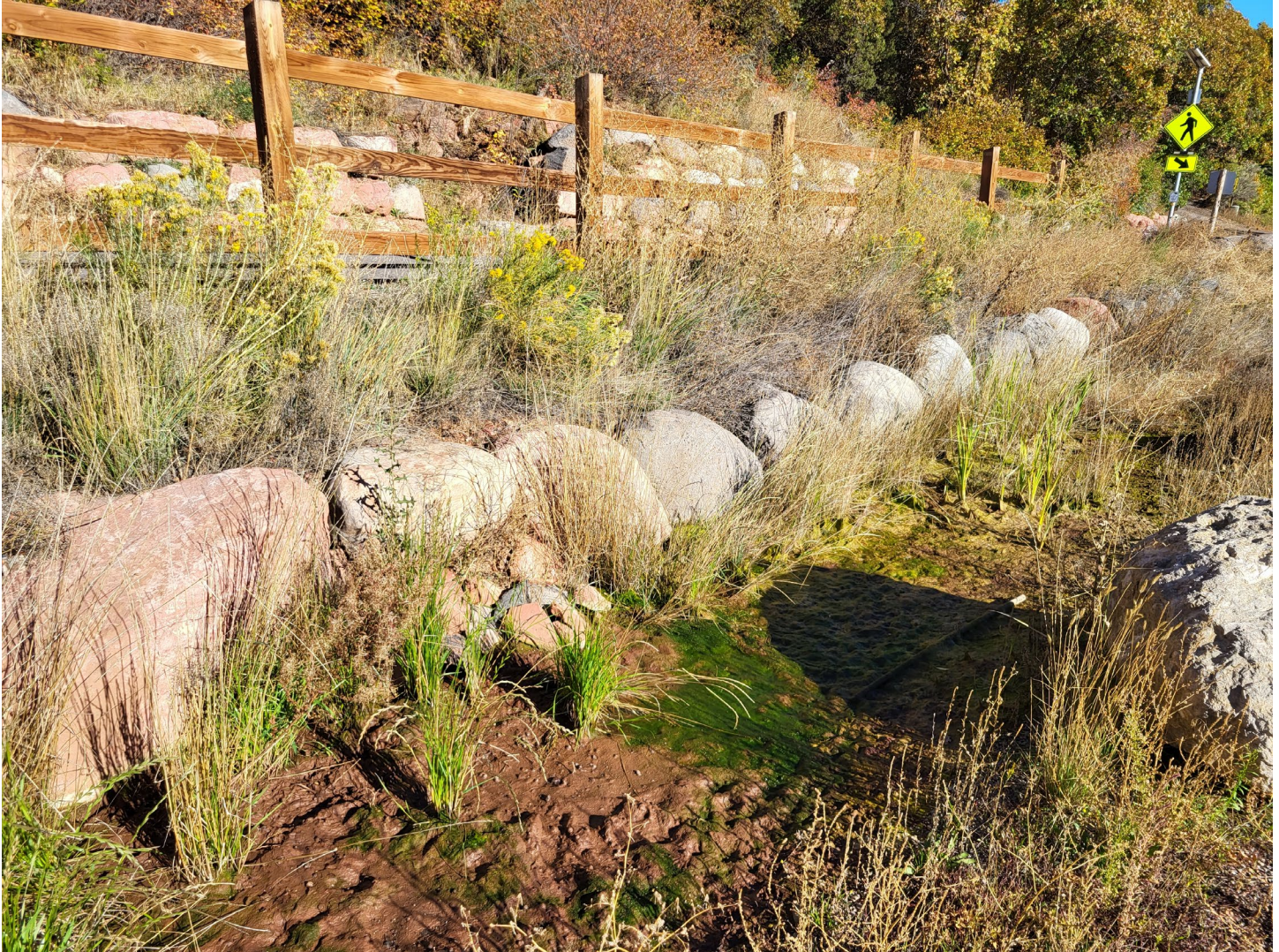
Photo – location #1 water from Thompson Glen Ditch seen down along CR 154 (photo taken 10/16/2023 just after ditch turned off for the season). Small culvert under Hardwick Bridge Trail is already getting clogged with sediment.
