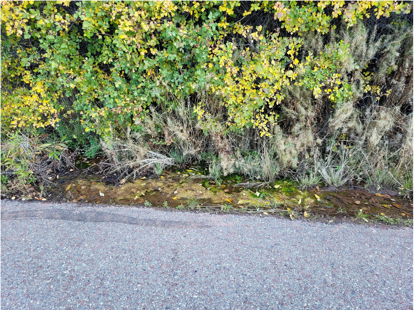
Photo – location #3 ditch water along shoulder of RGT
