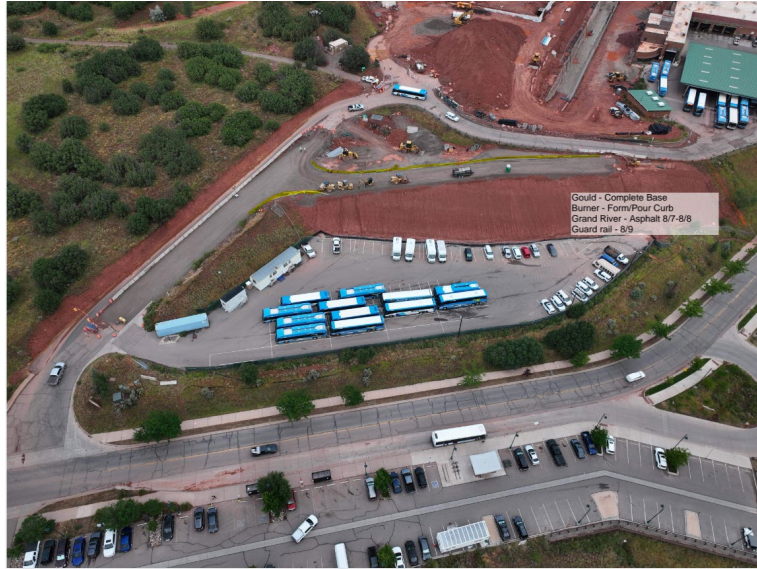
Paving of New Access Road
