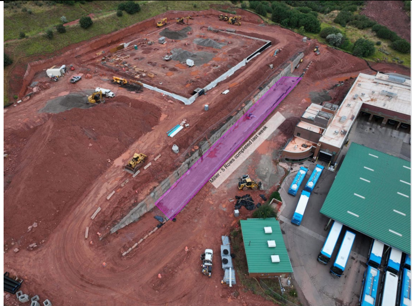
Ground prep for Fuel/Wash bay
