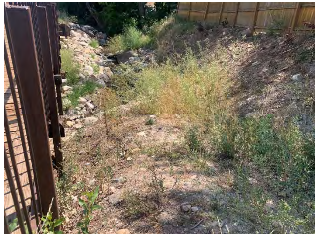
Figure 19 –View of slope to western bank of Sopris Creek.
