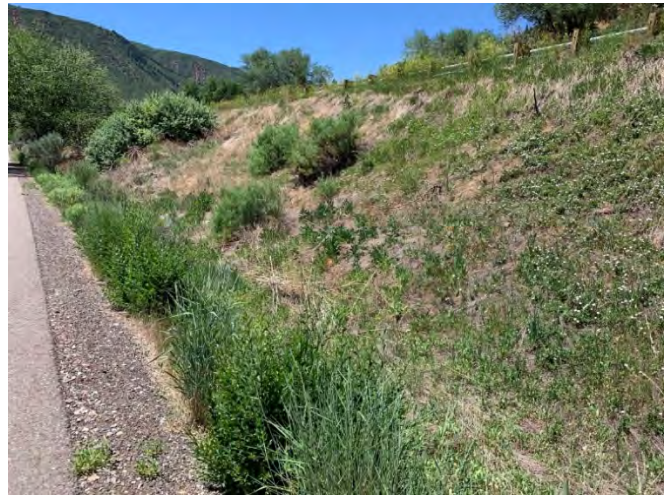
Figure 18. View looking NW at restoration Priority 4.
