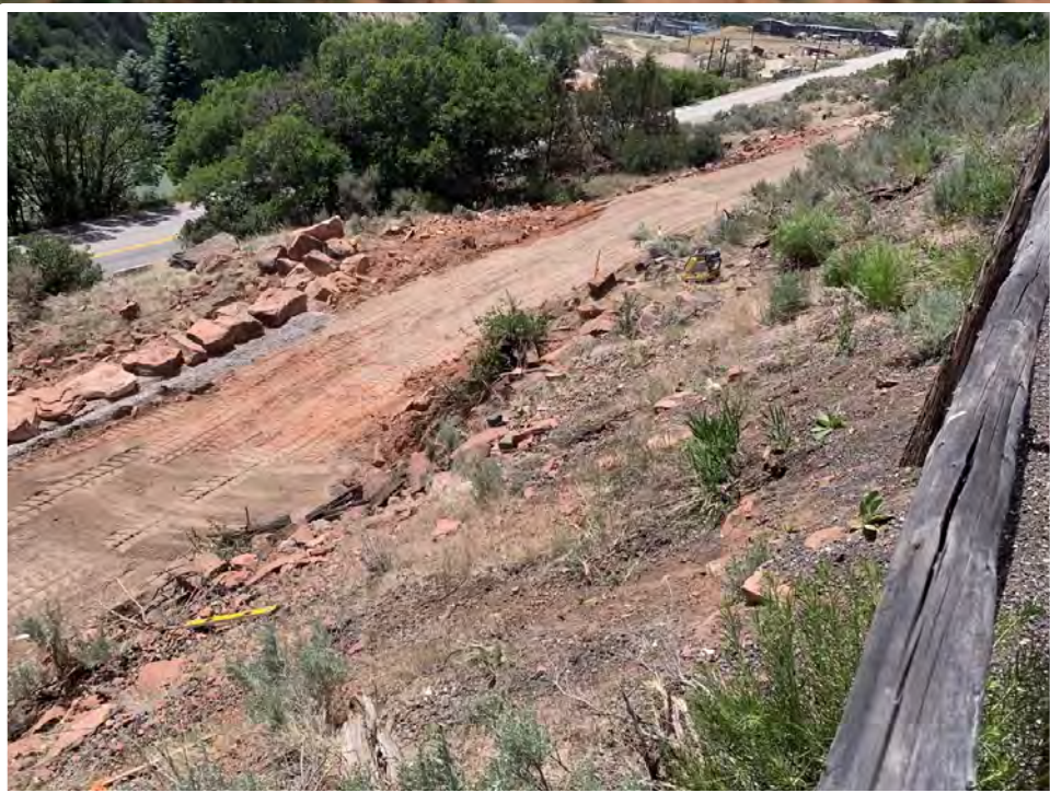
View looking NW at Restoration Priority Area 1 from Rio Grande trail. Establishing native grasses along the poorly vegetated bank using seed mix #4 will help prevent erosion and provide aesthetical and ecological benefits.
