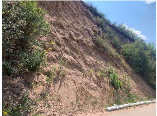
Figure 9 - View looking west (down valley) at priority area 1.
