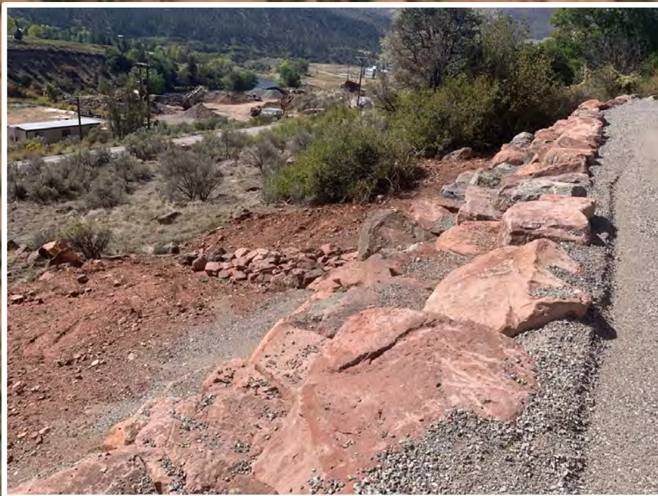
View Looking NW at Restoration Priority Area 1 for newly constructed trail. Bare soil areas should be seeded with seed mix #4 to provide quick establishment of native grasses to compete with noxious vegetation and to stabilize the soil.
