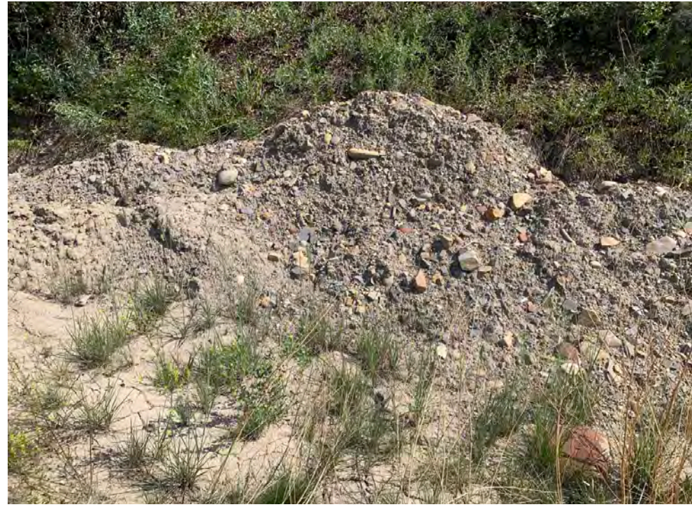
2. View significant impairment area along the south shoulder of the trail. Accumulated and piled fill material. Remove and seed area.
