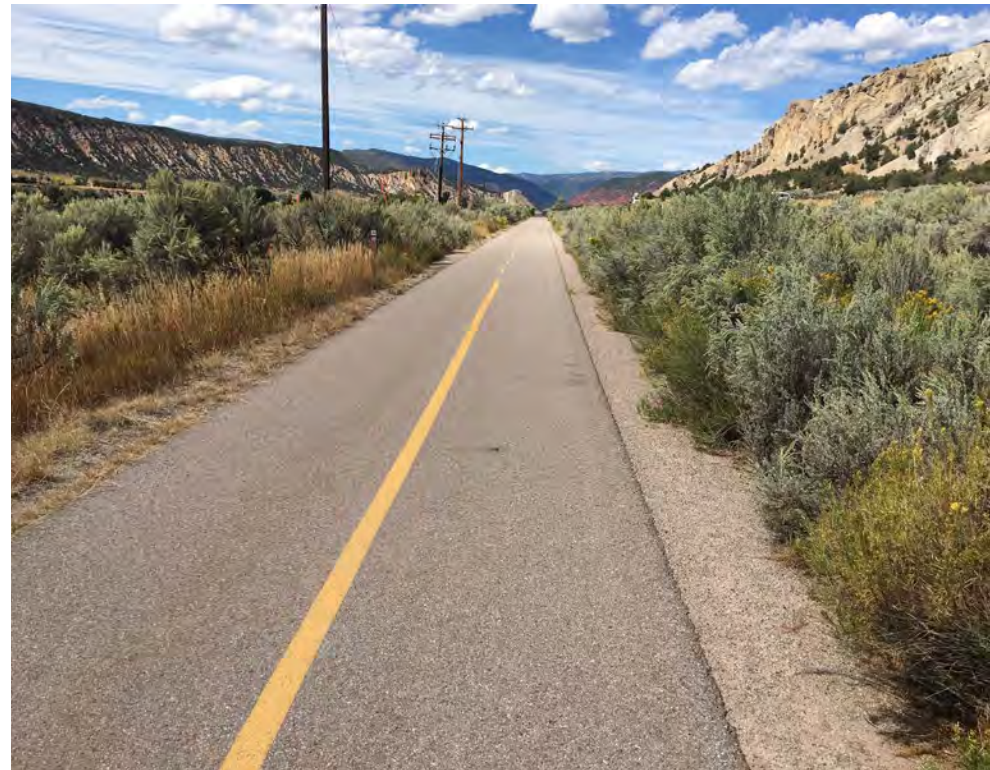
5. View looking NW at area of low impairment. Good establishment of native vegetation consistent with a sagebrush shrubland community.
