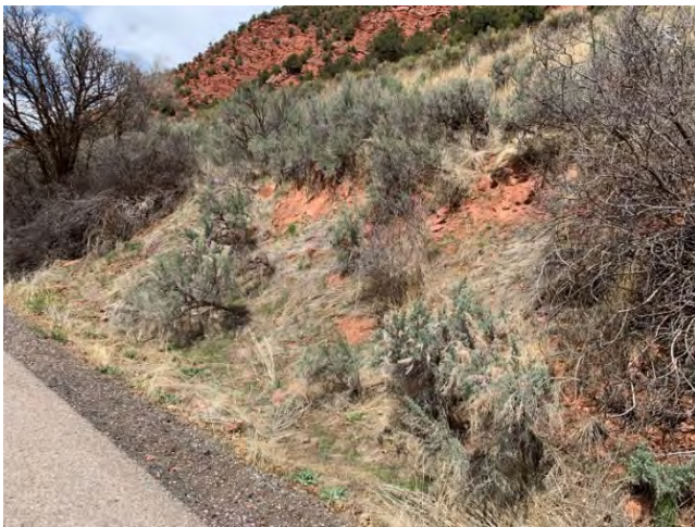
Figure 13. View looking NW at area of poor vegetation on steep slope
