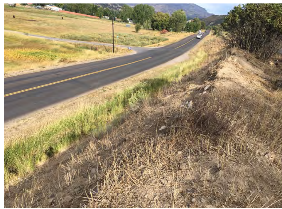
View looking east along restoration priority area 1, MP 374. Recommended restoration objectives include grading of the top of the slope to level out the unnecessary berm, amending soils as outlined in document and stabilizing slopes with Hydraulic erosion control product.
