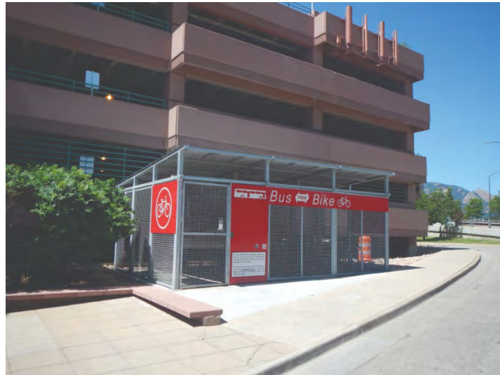
FIGURE 1. EXAMPLE OF BICYCLE STORAGE AT TABLE MESA PARK-N-RIDE, BOULDER
