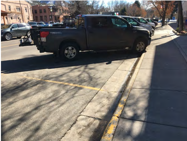
FIGURE 39. EXAMPLE OF FADED CURB PAINT ON COLORADO AVENUE
