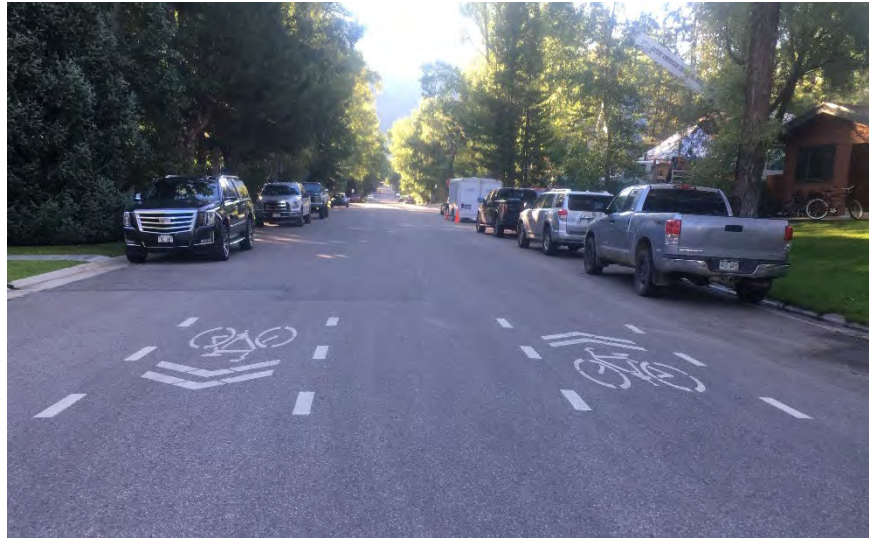
FIGURE 2: "SUPER SHARROW" PAVEMENT MARKING IN ASPEN, CO INDICATES PRIORITY & POSITIONING FOR BICYCLISTS ON SHARED ROADWAY.
