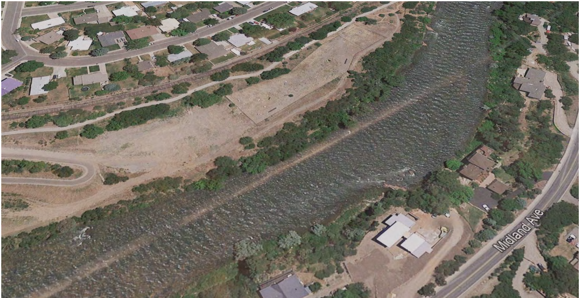
FIGURE 6. RIO GRANDE CORRIDOR BRT: EXISTING
