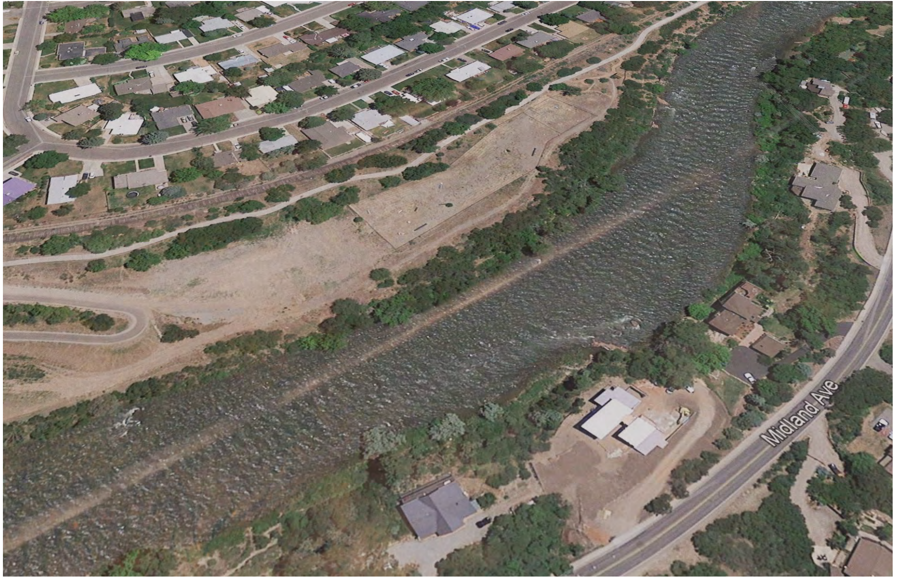
FIGURE 57 - RIO GRANDE CORRIDOR BRT EXISTING
