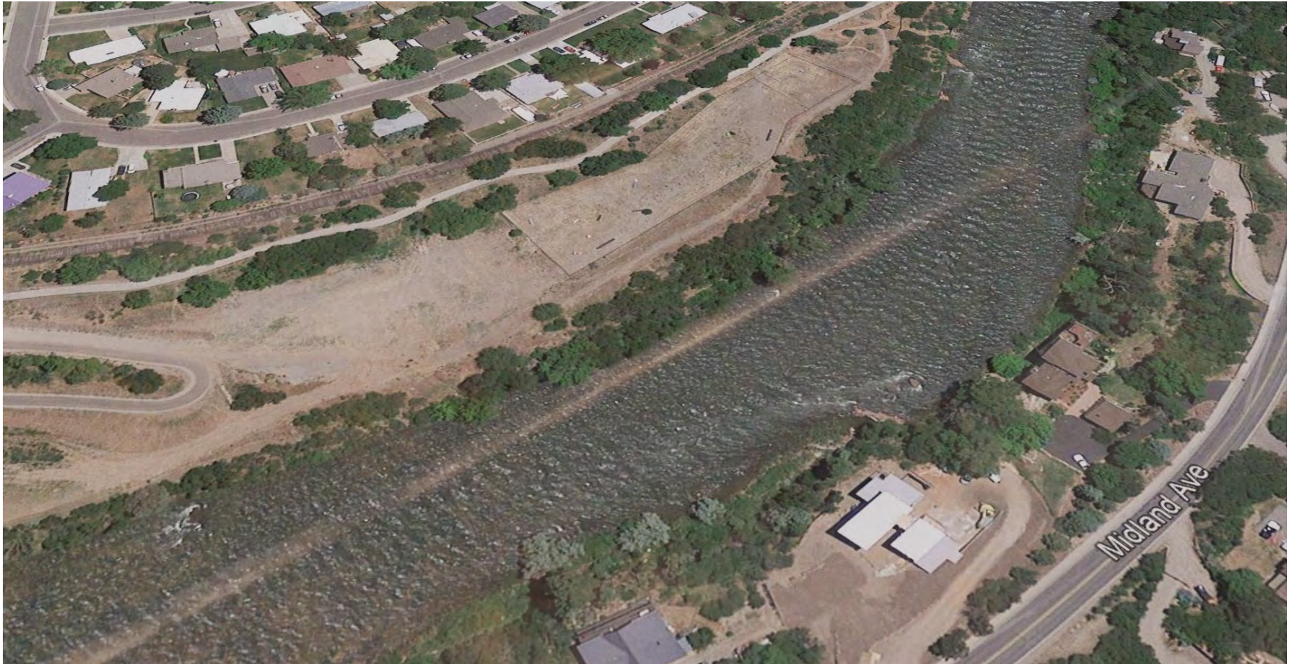
FIGURE 23. RIO GRANDE CORRIDOR BRT: EXISTING
