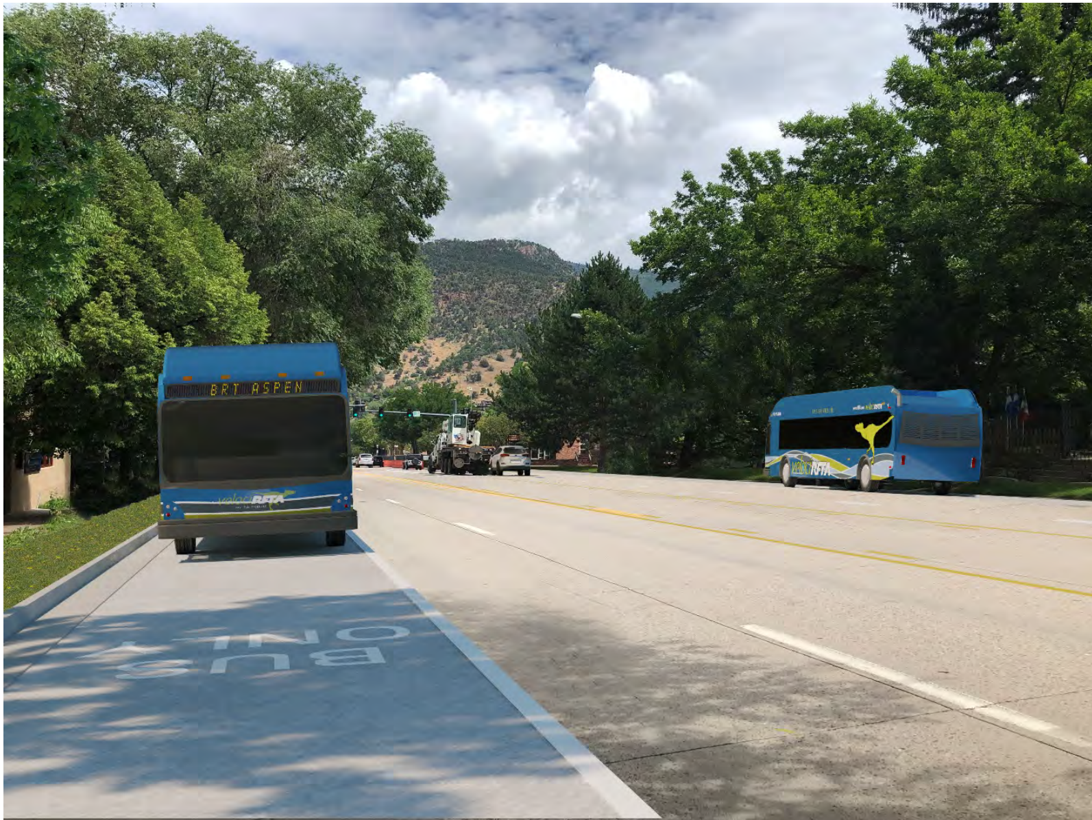
FIGURE 19. GRAND AVENUE SEMI-DEDICATED BRT LANES THAT ALLOW RIGHT TURNING VEHICLES
