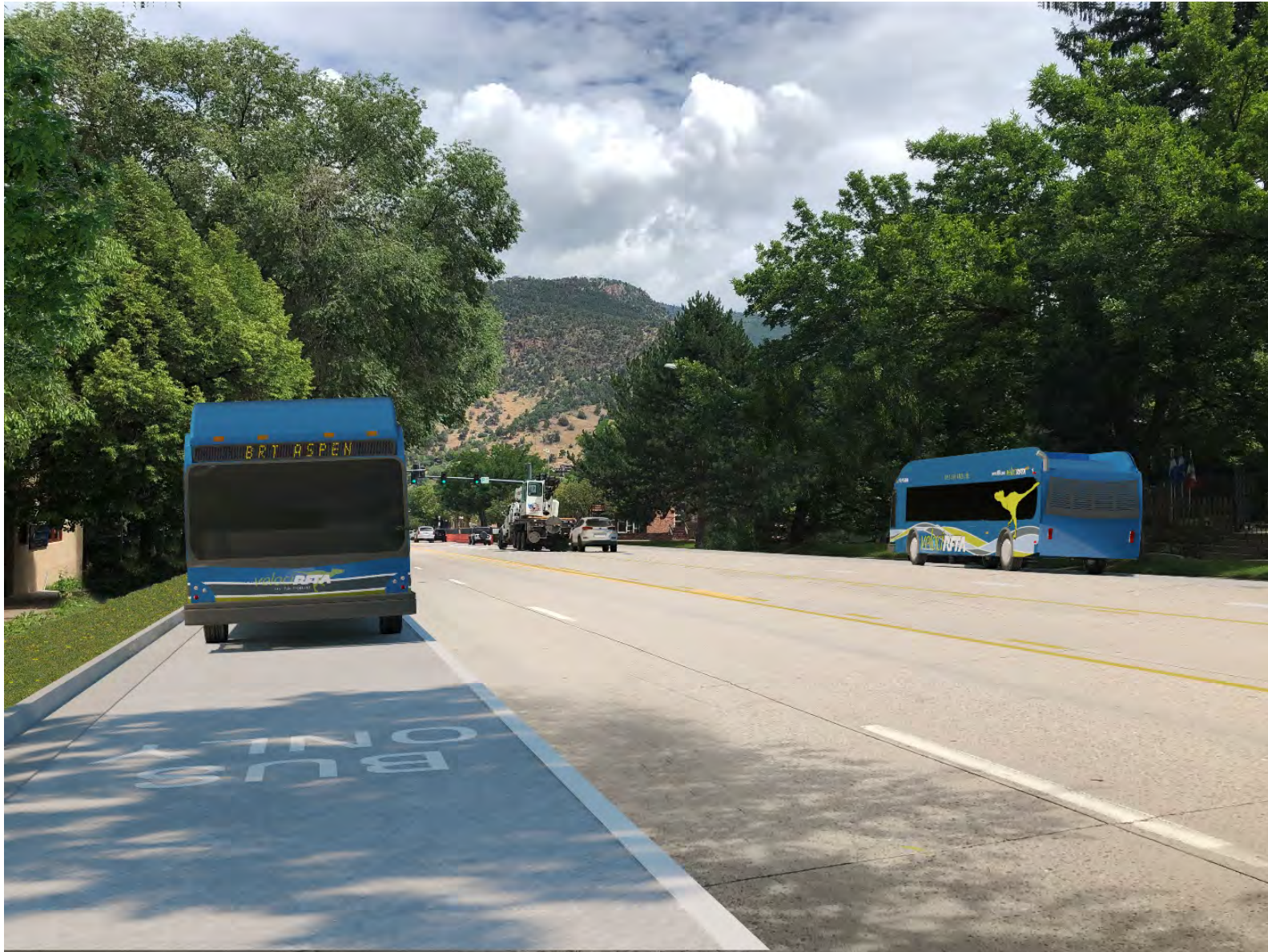
FIGURE 51 - GRAND AVENUE SEMI-DEDICATED BRT LANES THAT ALLOW RIGHT-TURNING VEHICLES
