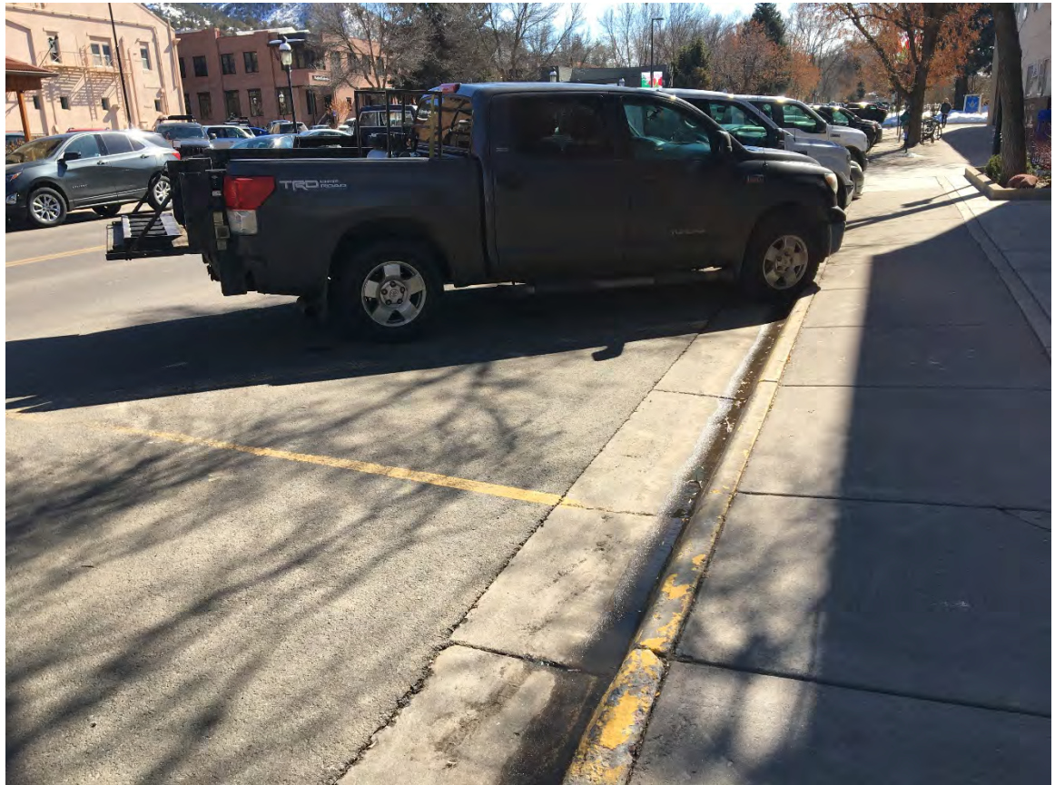
Example of partially visible yellow paint on a curb on Colorado Avenue.
