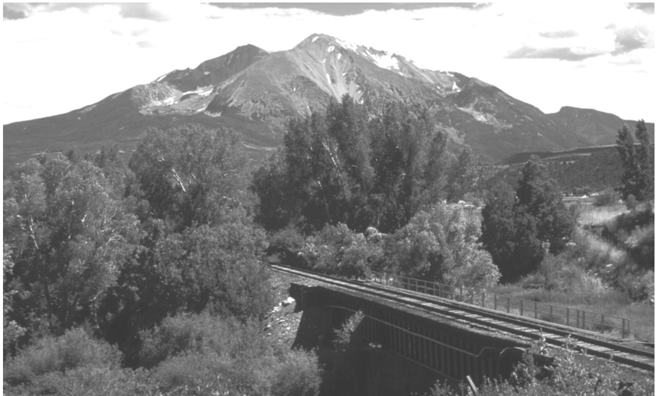
Figure III-15, below: Rail trestle with Mt. Sopris behind – Downvalley from Carbondale
