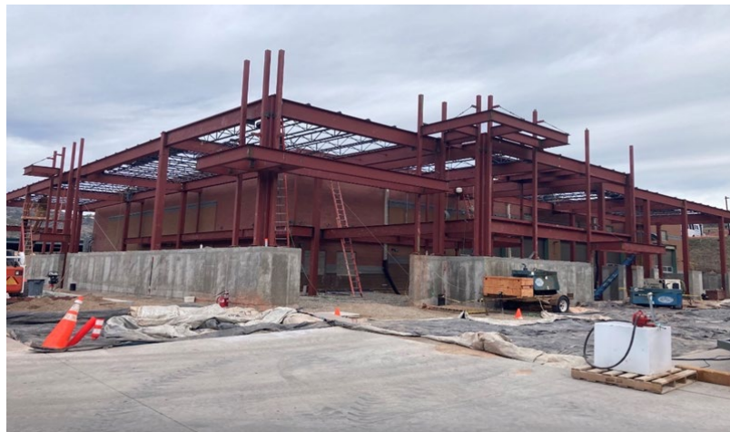
Steel being set at the Westside of the GMF
