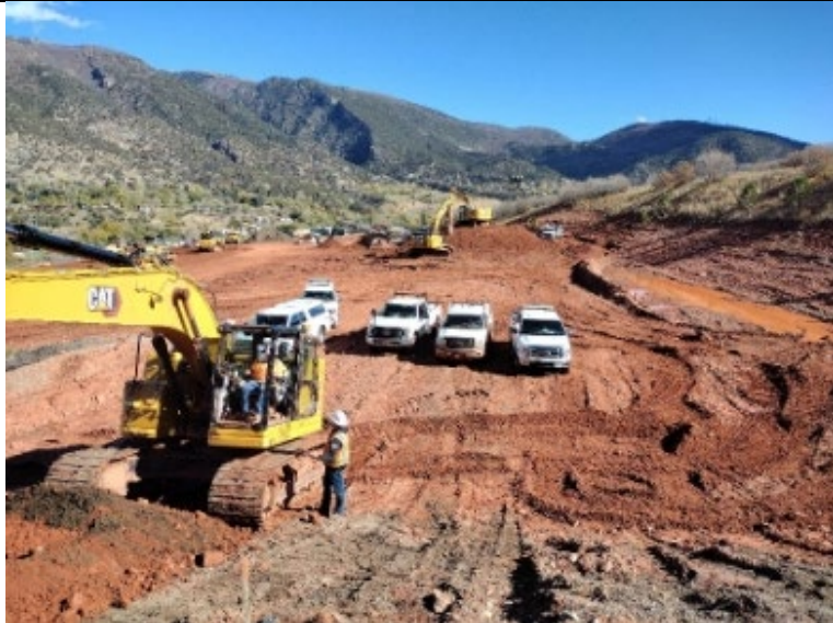
Grading and Soil Processing at GMF for Phase 3, 4, 5 and 7
