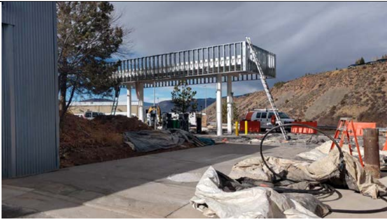
New Fuel Island and Canopy
