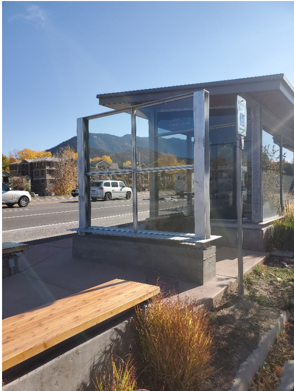
New Windscreen Installation
