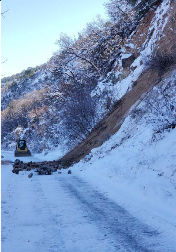
Rock scaling along Rio Grande Trail
