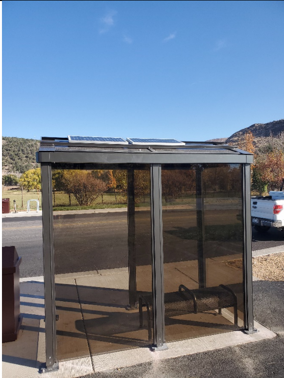
New Shelter Installation
