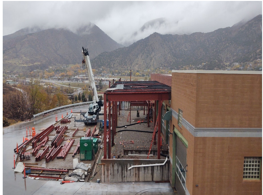
Steel being set at the Westside of the GMF
