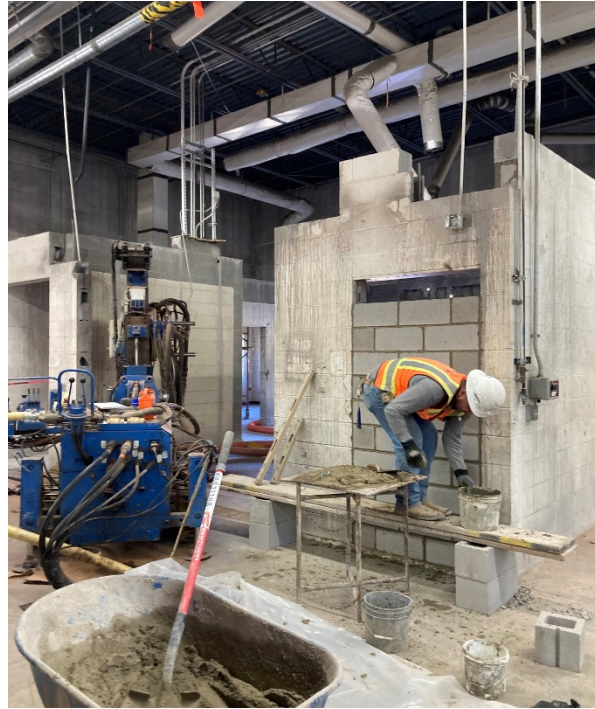
Masonry work happening inside the GMF
