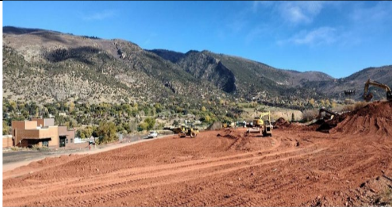
Demo and Grading at GMF for Phase 3, 4, 5 and 7
