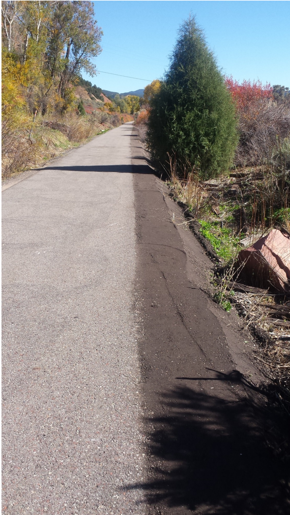
Photo – after shoulder repair, no more lip...instead a good 2' shoulder!
