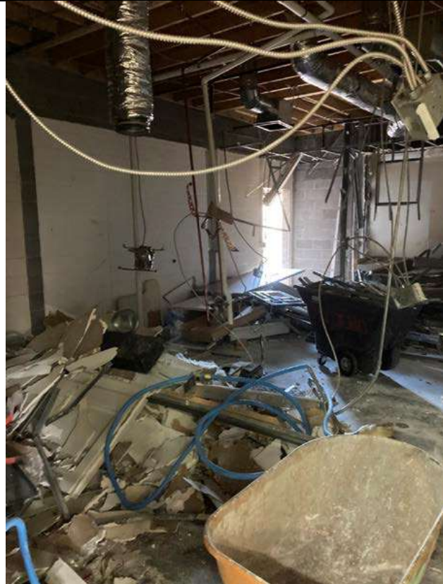
Interior remodeling at the GMF
