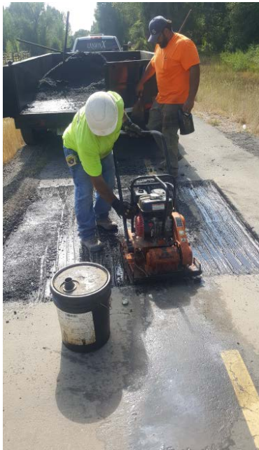
Rio Grande Trail Pavement Repair
