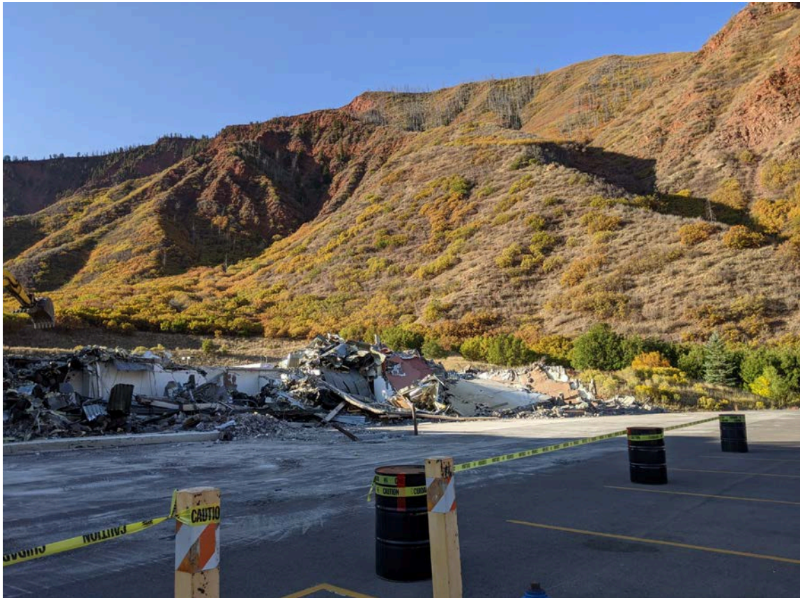
Demolished West End of Glenwood Maintenance Operations Center
