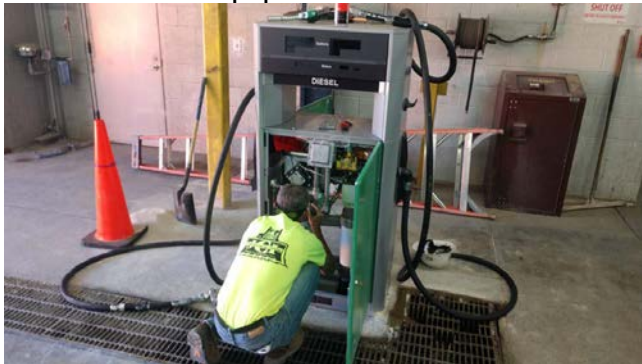
Interior Fuel Pumps being installed
