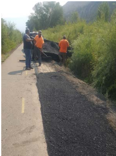
Rio Grande Trail Pavement Repair
