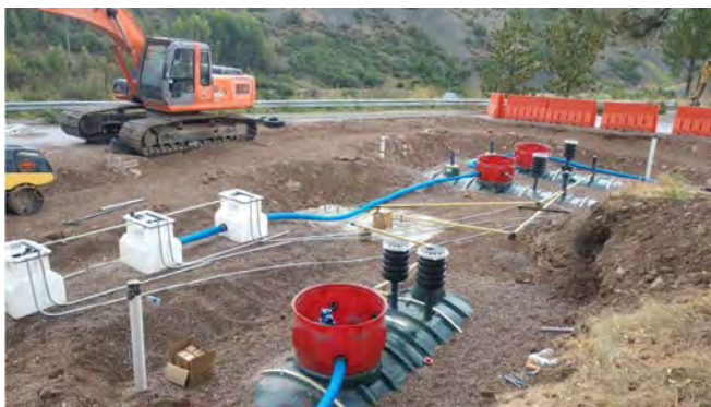
AMF Fuel Farm Installation
