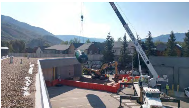
New Oil Tank being lowered in place
