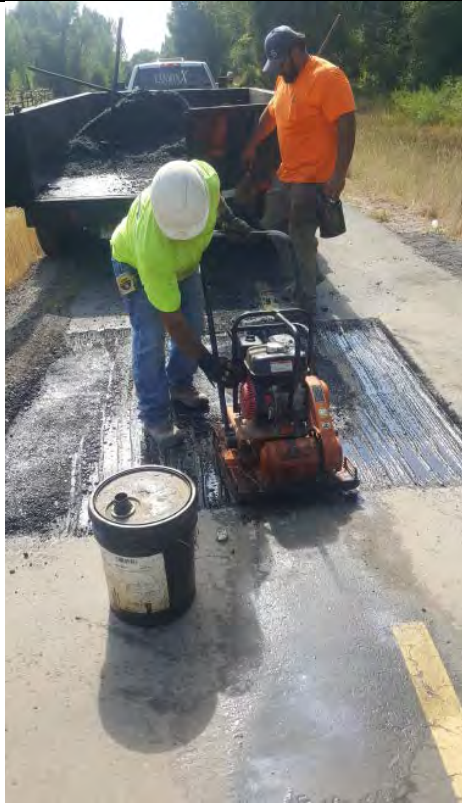
Rio Grande Trail Pavement Repair
