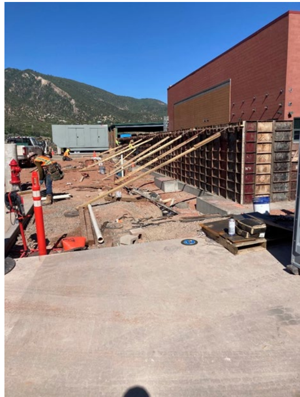
Concrete forming work at the GMF
