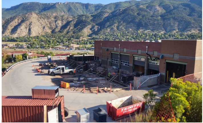
Foundation prep at the west side of the GMF
