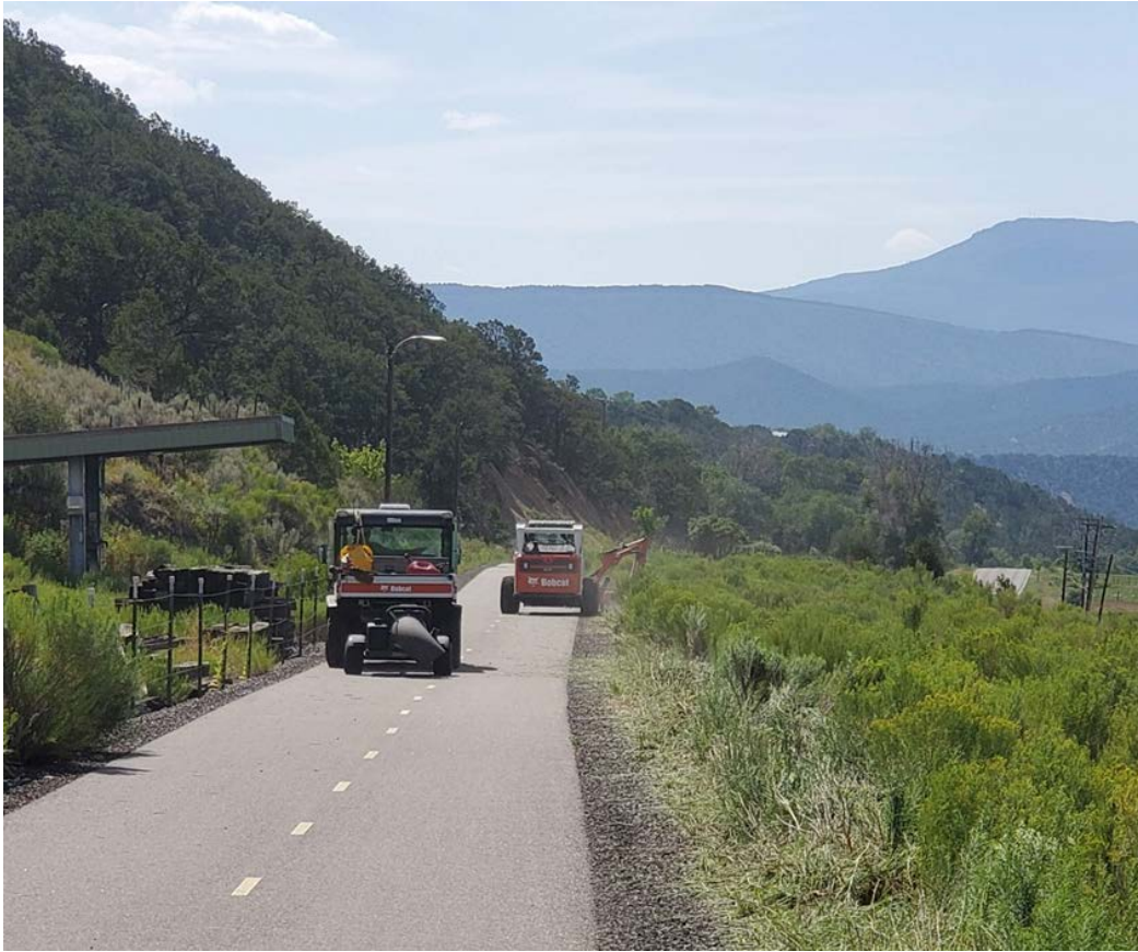
Photo 1 – Mowing the shoulder with the flail mower and blowing the cut grass/debris off the trail, immediately following the mower.
