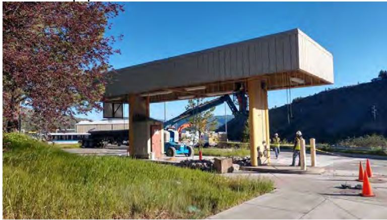
Fueling Canopy demolition
