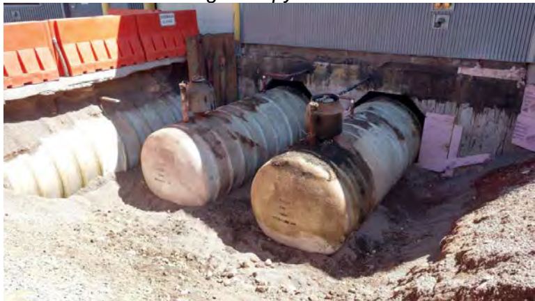
Removal of underground tanks
