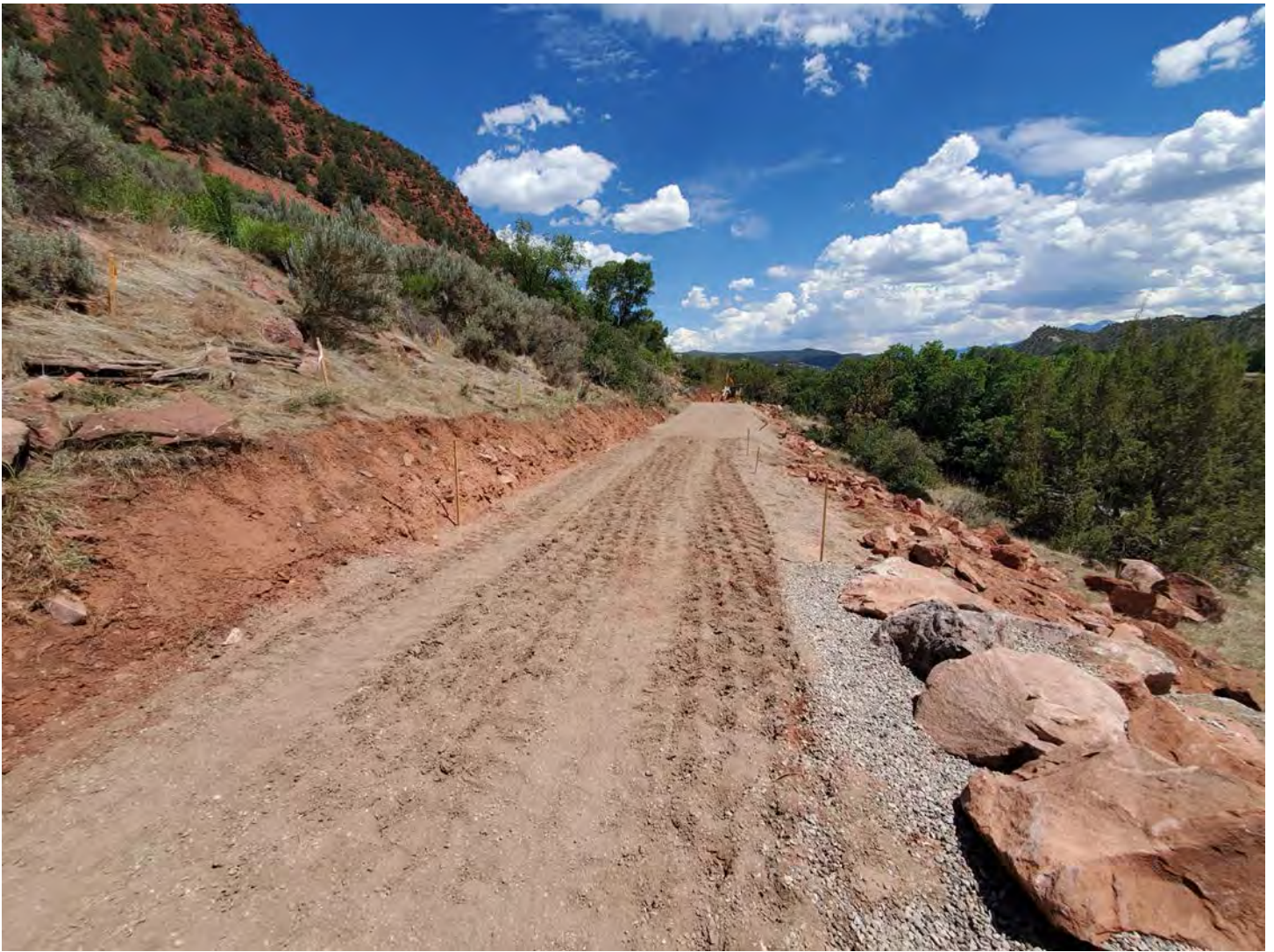
Photo 4 – Safe Routes to School “Riverview Trail” construction progress.
