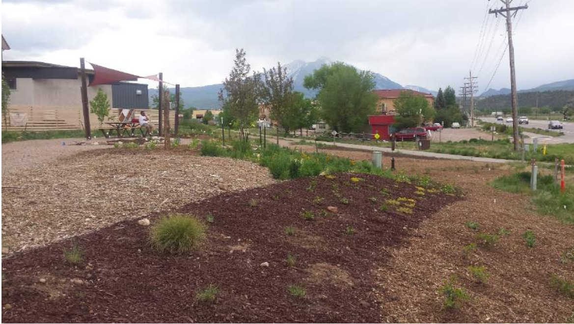
DeRail Park – Shade Sail, picnic table, and landscaping installed!
