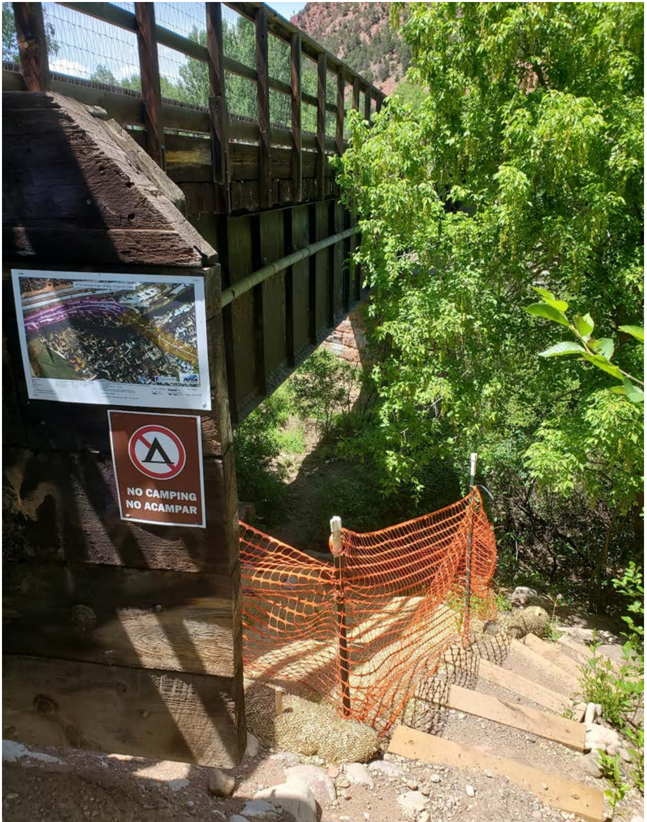
Photo 3 – Improved “social trail” down to the Roaring Fork River. ROW Map posted to educate users of property boundaries. Revegetation efforts on the steep slope; grass seed and erosion control BMPs.
