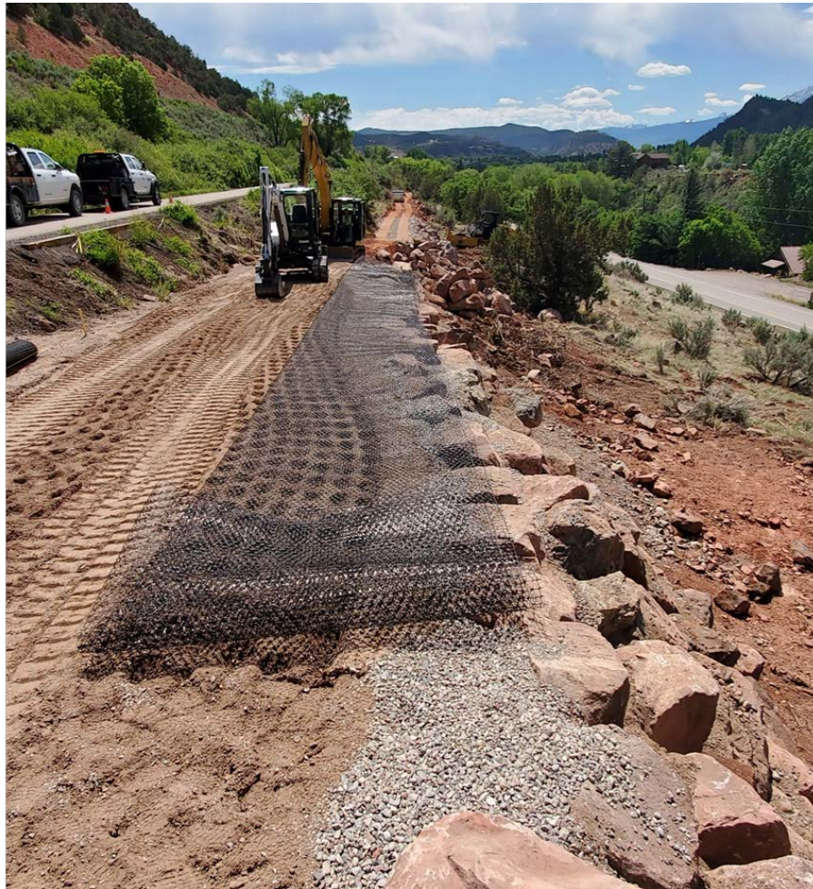
Photo 2 – Riverview Trail construction
