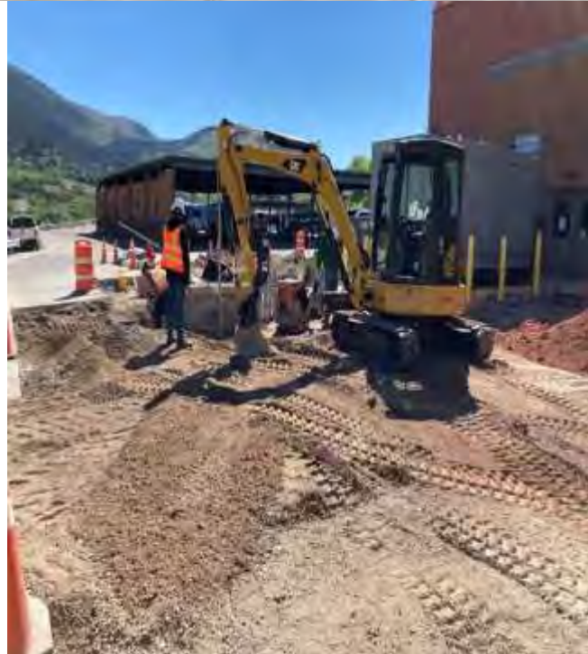
GMF Phase 2 Construction Activity
