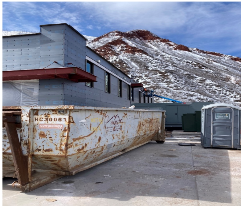
Exterior siding being attached
