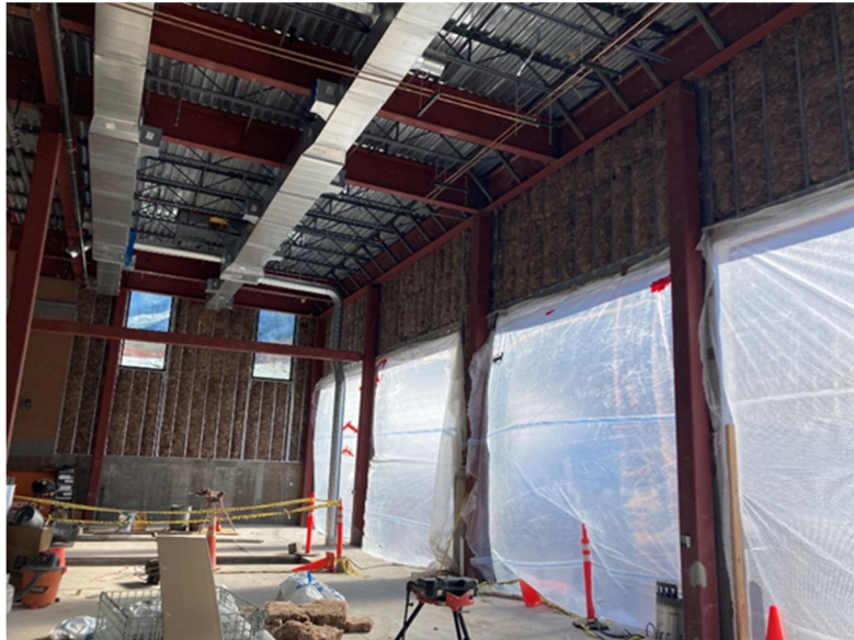
Expanded garage area
