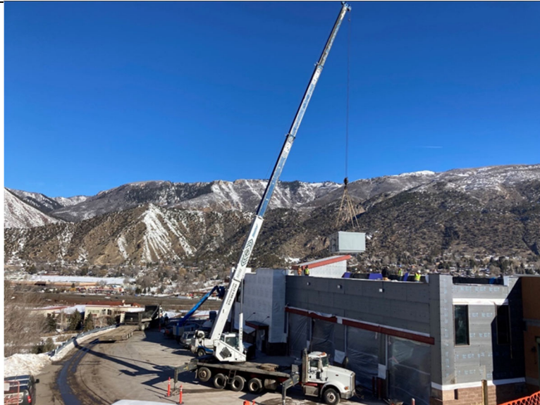
Rooftop mechanical units being set
