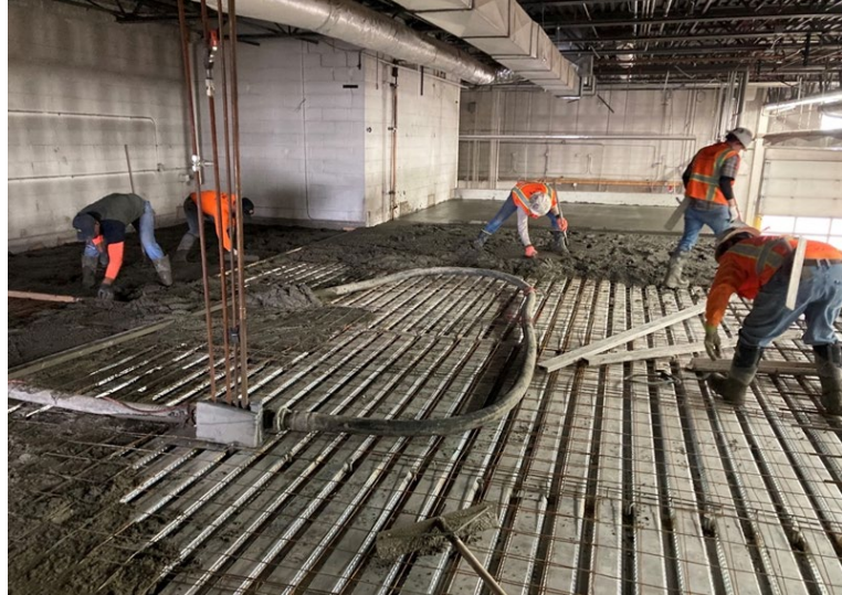
Concrete being poured at the mezzanine area of the GMF
