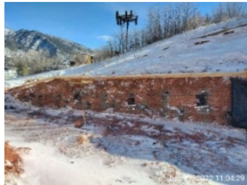
South wall construction
