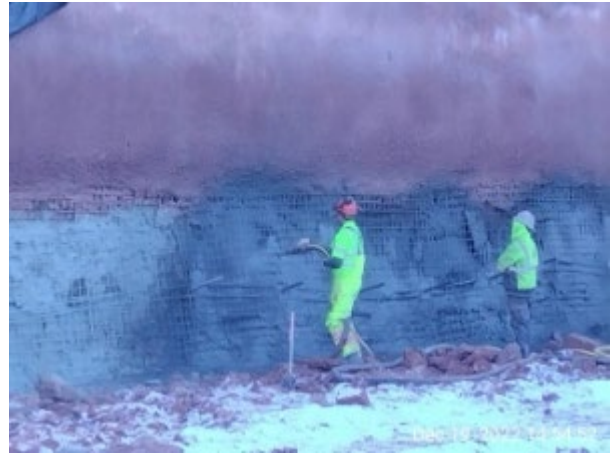
South wall construction
