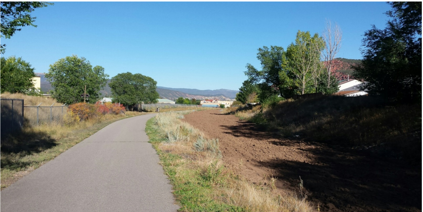
Photo 1 – Dirt through the Town of Carbondale. The dirt will be seeded with a native grass and wildflower mix and covered with straw before winter.
