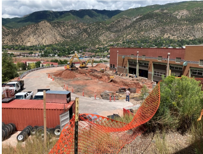
Excavation at the west side of the GMF
