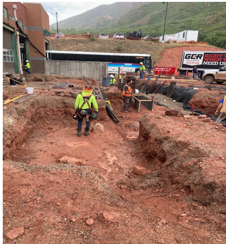
Concrete forming work at the GMF
