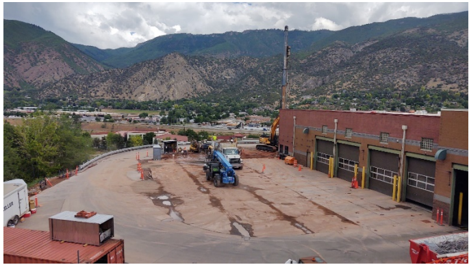
Compaction grout columns being installed
