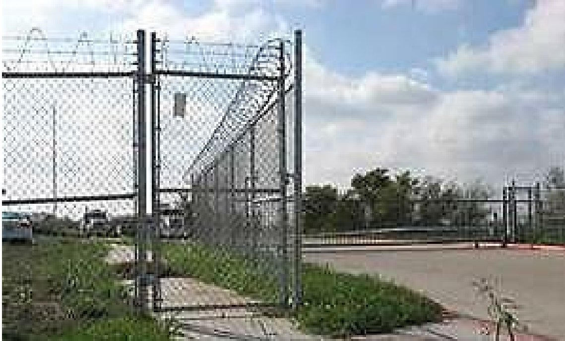
Exhibit 9 - Chain link Security Fence pedestrian gate
