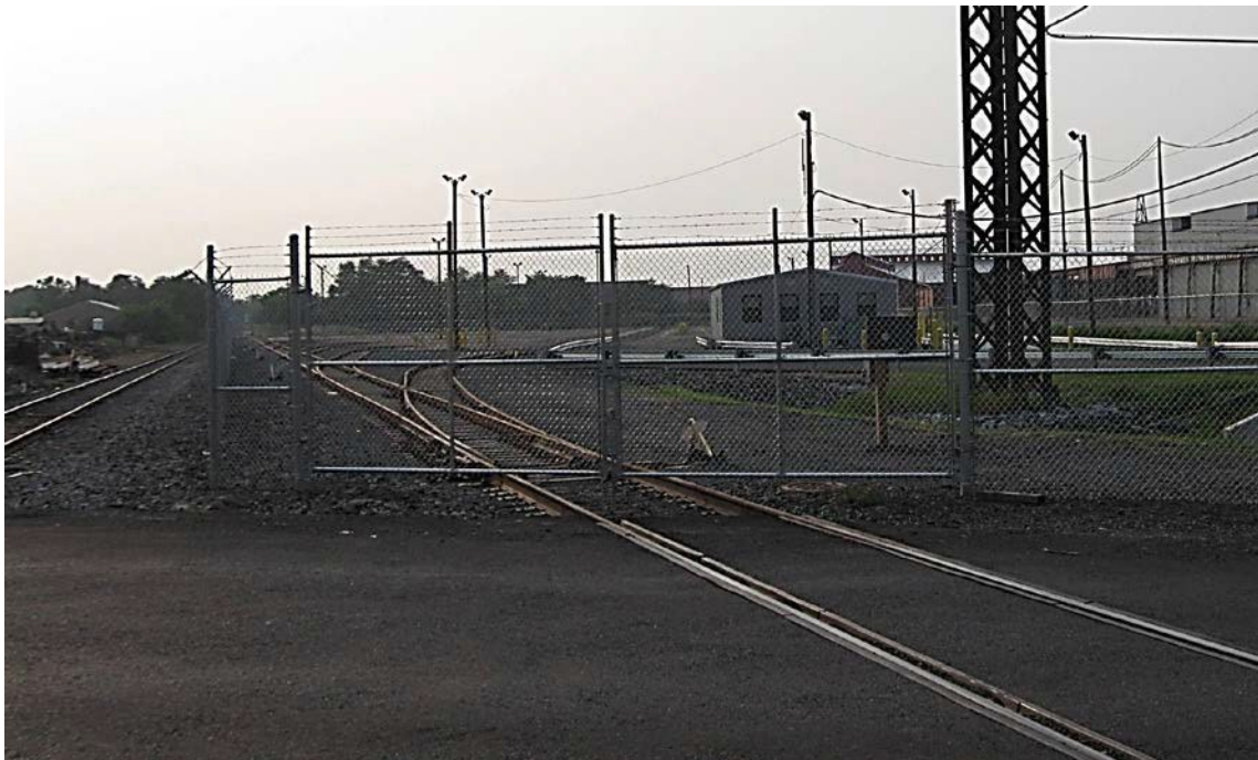
Exhibit 10 - Chain link Security Fence double swing gate in a track application
