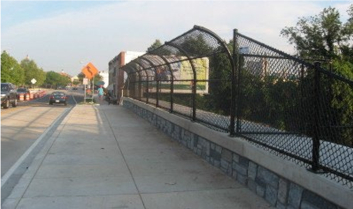
Exhibit 30 – Overhead Bridge Fencing using Decorative Finish chain-link product.
