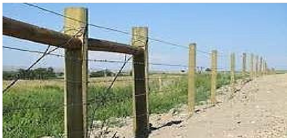
Exhibit 3 – Multi-strand Barb Wire Right-of-way (Range) Fence
