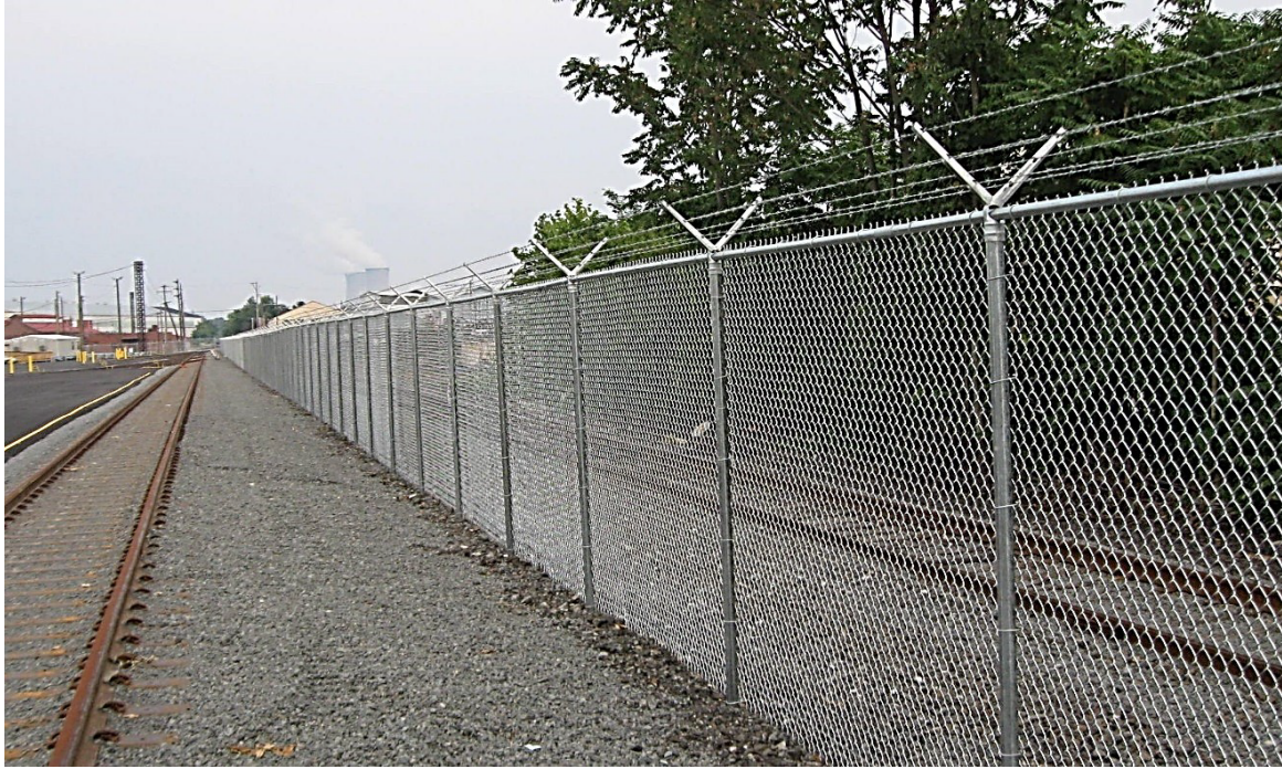
Exhibit 7 - Chain link Security Fence with 6 strand barbed wire on dual arms
