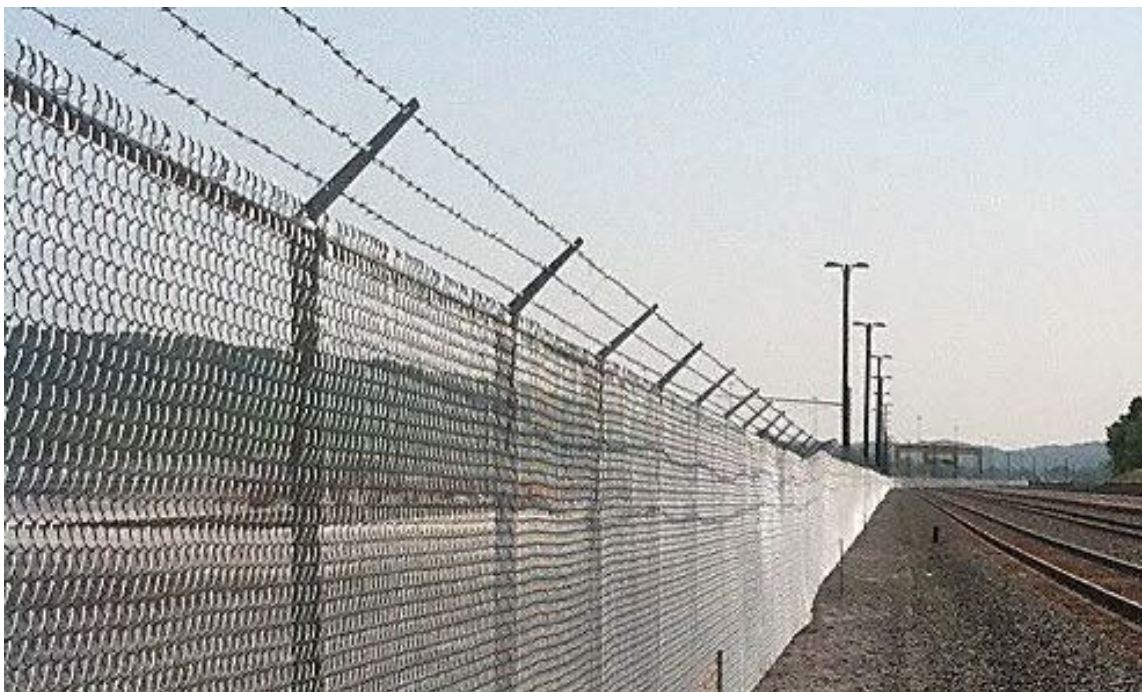
Exhibit 6 - Chain link Security Fence with 3 strand barbed wire on single arm
