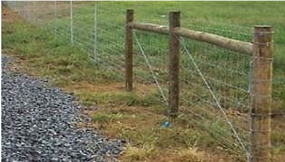
Exhibit 1 – Woven Wire Right-of-way Fence
