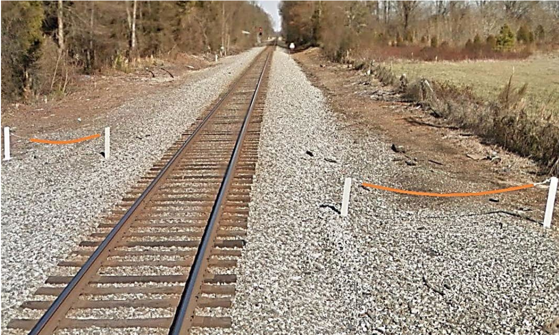
Exhibit 17 - Cable Right-of-way Barrier Gate
