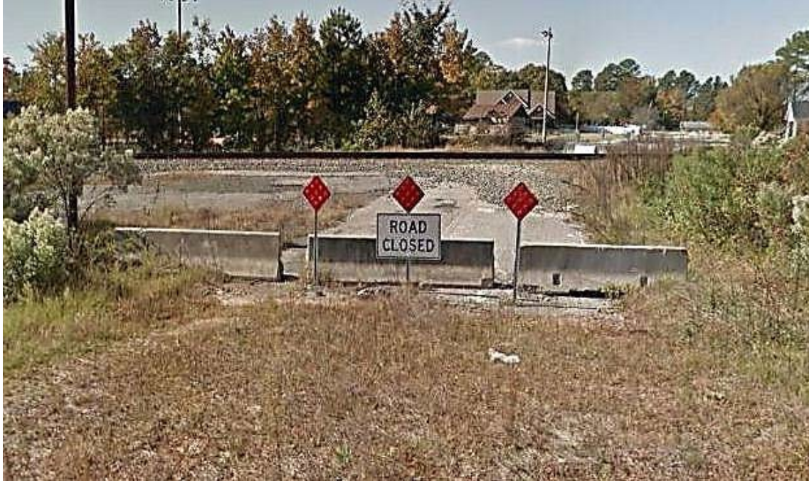
Exhibit 14 - Concrete 'Jersey' Barrier
