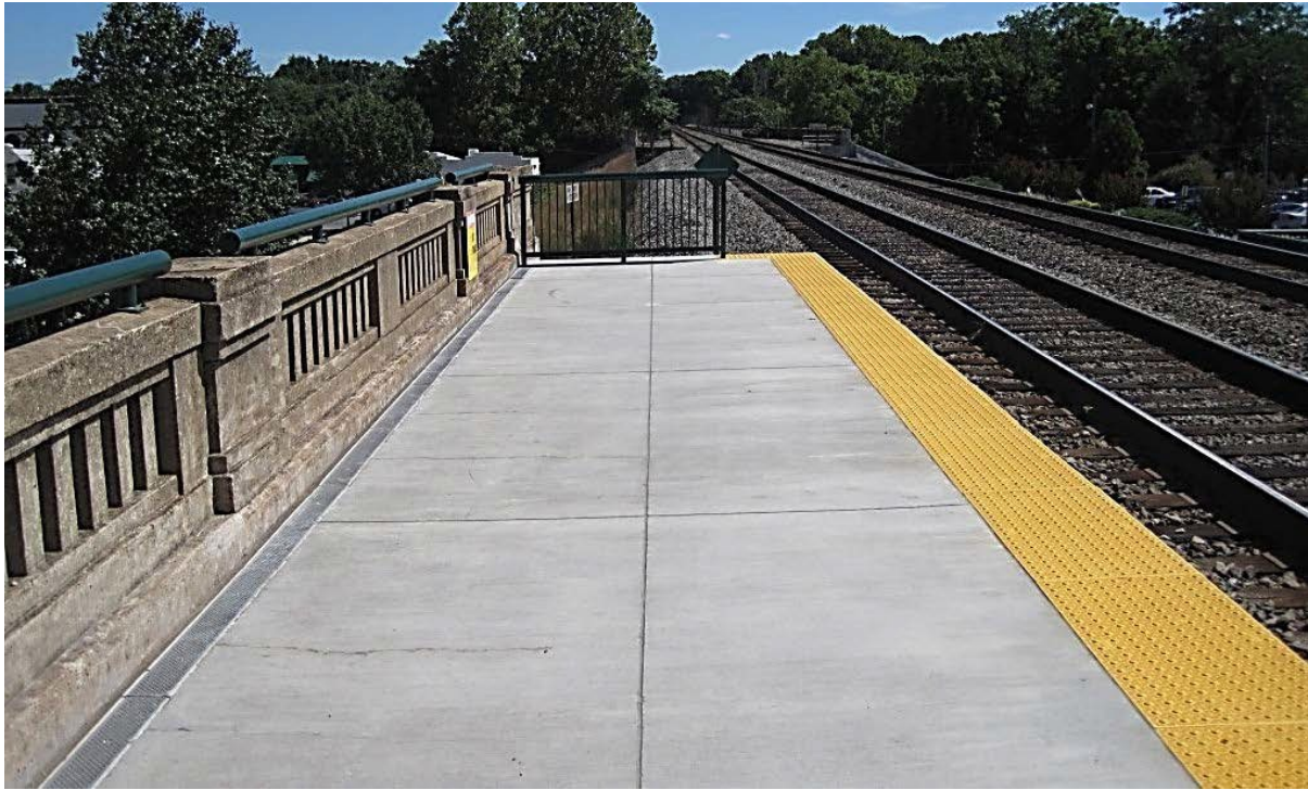
Exhibit 22 - End of Platform Barrier – note setback from platform edge.
