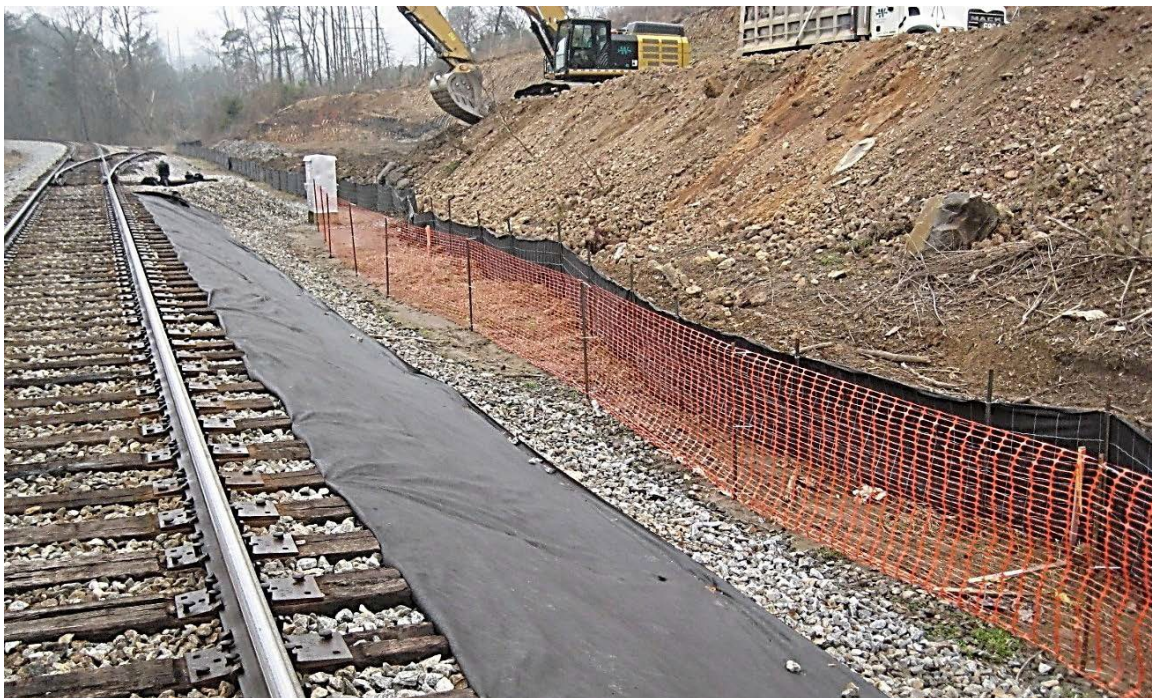
Exhibit 13 - Temporary Barrier Fence
