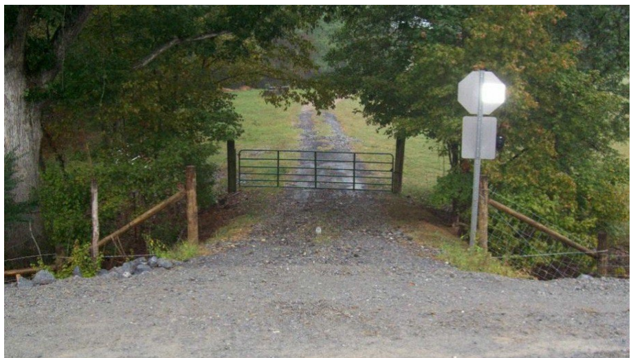
Exhibit 2 – Offset Right-of-way Fence Swing Gate (viewed from track zone)
