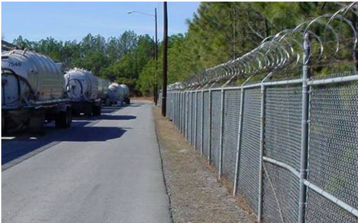
Exhibit 8 - Chain link Security Fence with 3 strand barbed wire and barrier tape
