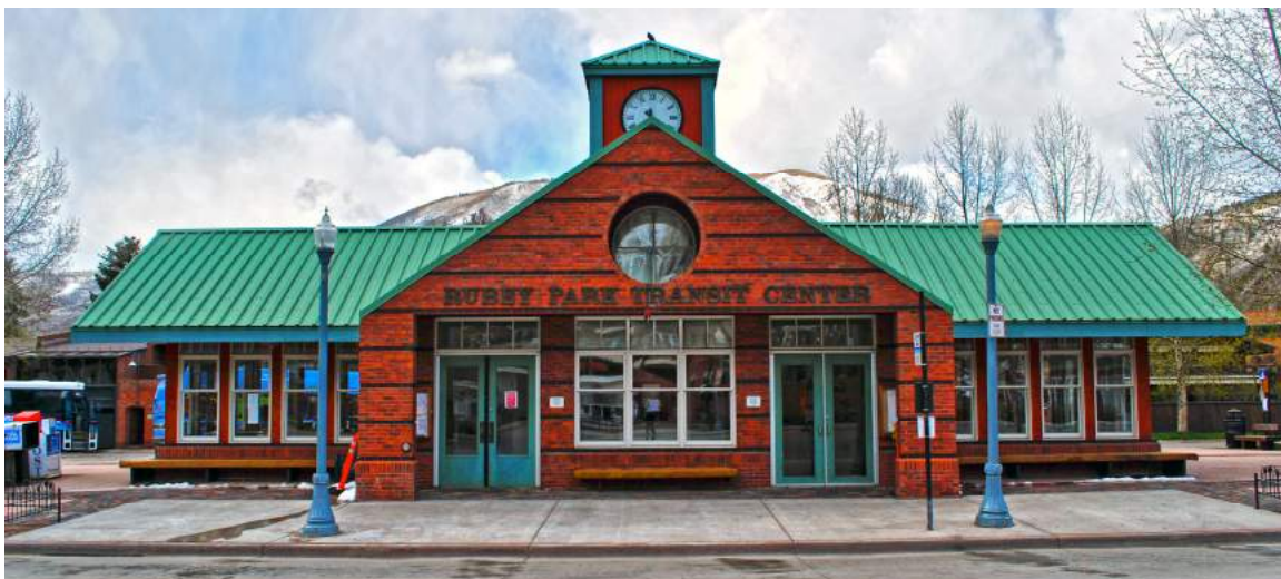
Built over 30 years ago, Aspen’s Rubey Park Transit Center will be remodeled in 2015.
