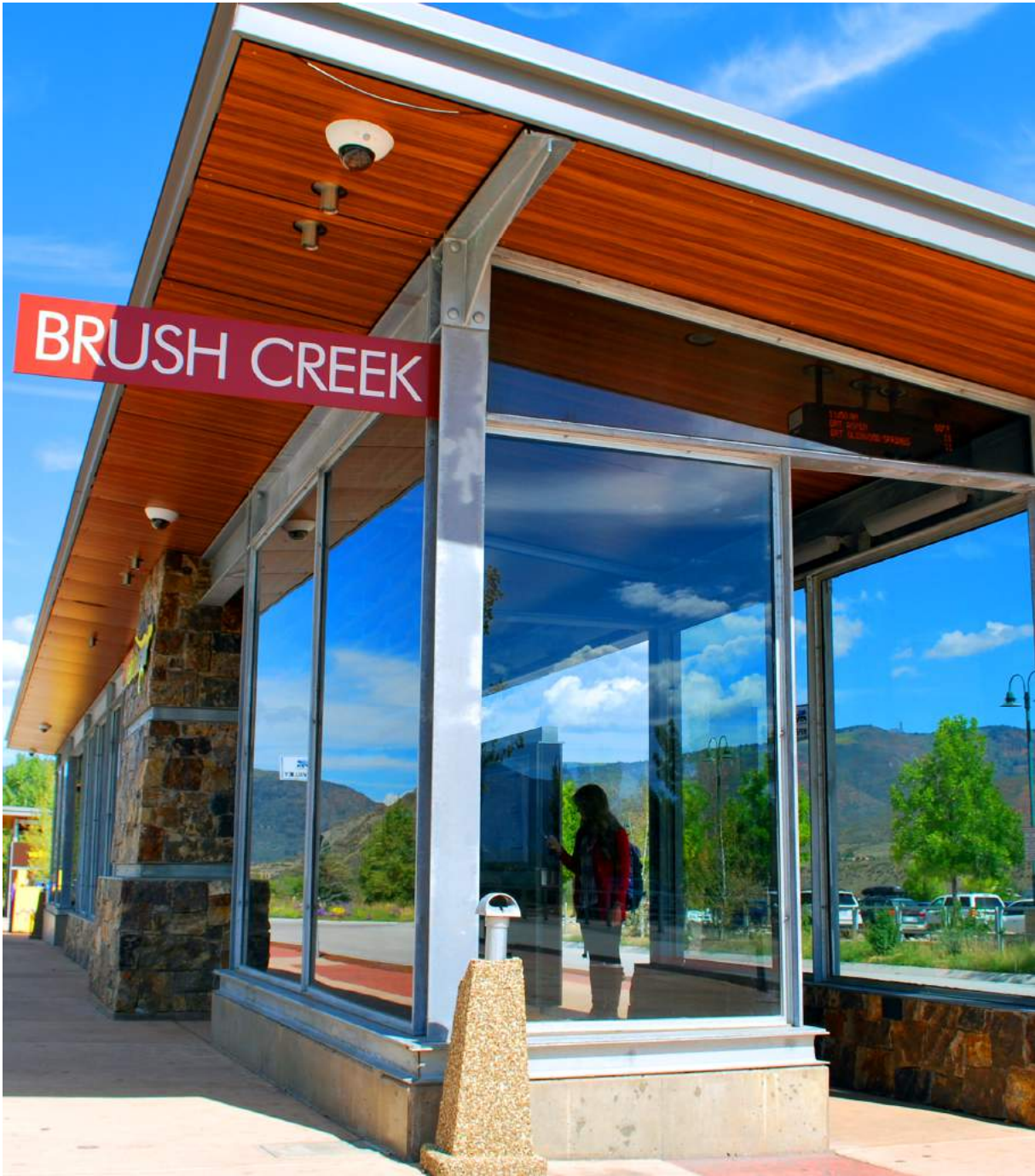
Brush Creek is one of thirteen new VelociRFTA Bus Rapid Transit stations along Highway 82.
