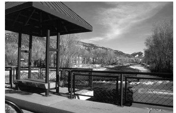
BASALT – MIDLAND AVENUE BRIDGE
