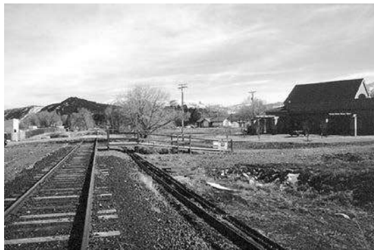
CARBONDALE – EXISTING RAIL ALIGNMENT
