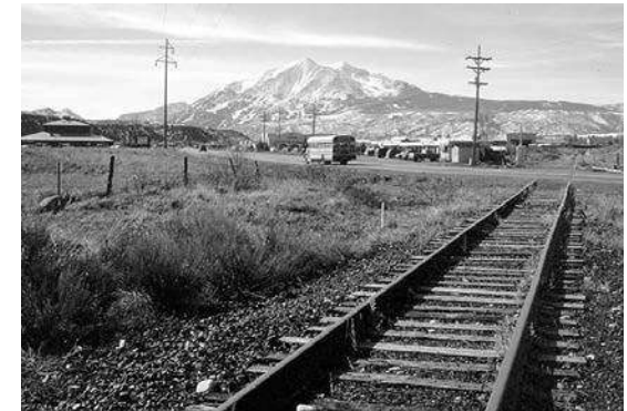
CARBONDALE – HIGHWAY 133 RAIL CROSSING
