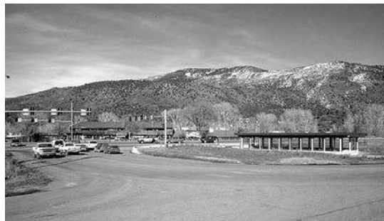
EAGLE COUNTY – PEDESTRIAN UNDERCROSSING AT EL JEBEL
