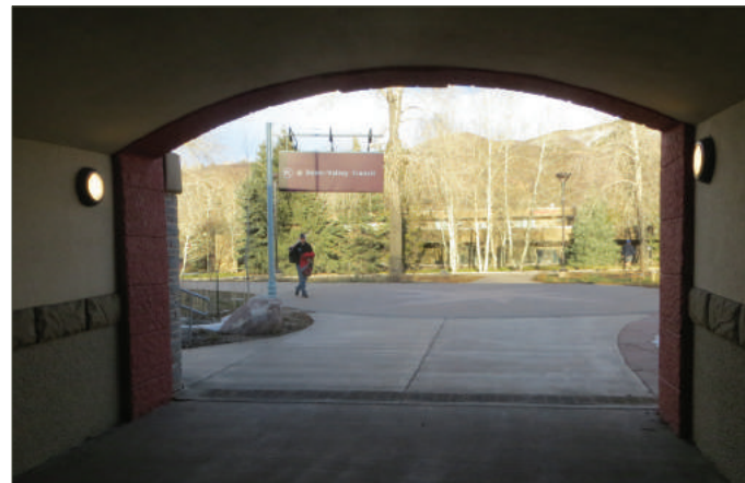
Figure 2.2: Bicycle and Pedestrian Underpass - Aspen
