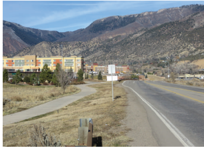
Figure 2.11: Shared Use Path along Roadway - Glenwood Springs
